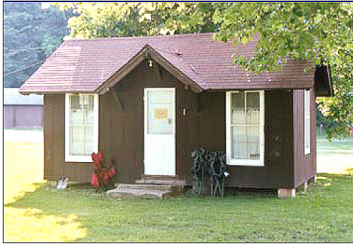
Figure 3. One of 10 cabins constructed by the CCC at the group camp area.
