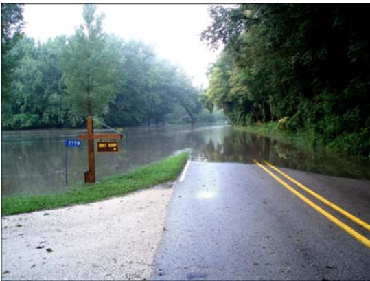
Figure 16c. Des Moines River floods park road in August of 2007.
