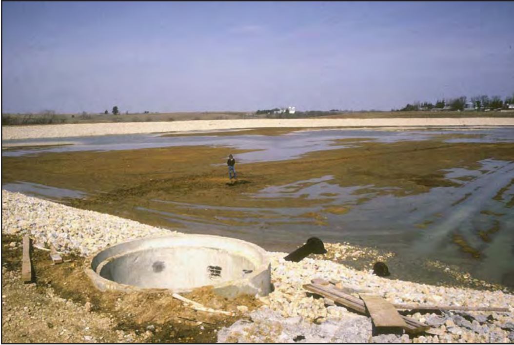
Figure 12-3. City of Garnavillo lagoon after sinkhole failure.
