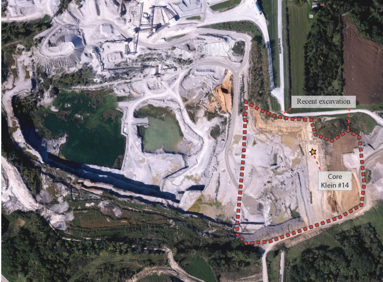
Figure 1. 2013 aerial photo of the Klein Quarry. Recent expansion operations to the southeast is outlined in red. Core sample ‘Klein #14’ will be available to the field trip attendees for study and is described in this guidebook.
