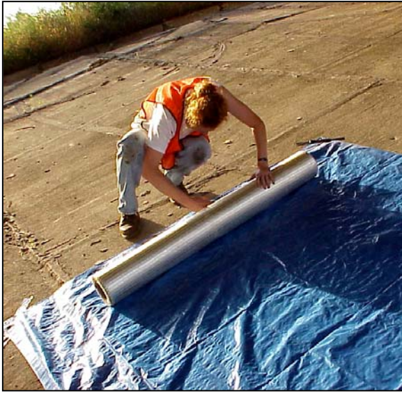
Figure A.18 Use a tarp or other protective cover to lay out the fiber.
