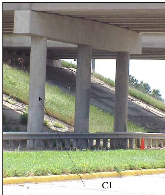
Figure 3.3 View of C1 prior to the FRP wrap installation.
