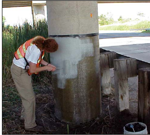
Figure A.34 Roll on the topcoat with a long nap roller.
