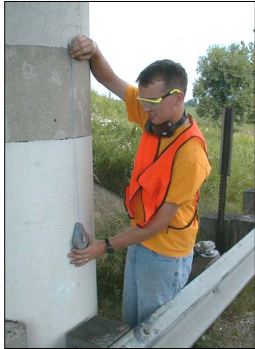
Figure 3.17 Use of a “plum-bob” to position the template.
