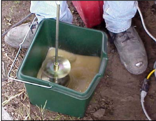
Figure A.13 Mix the primer's main agent and hardener for three minutes.
