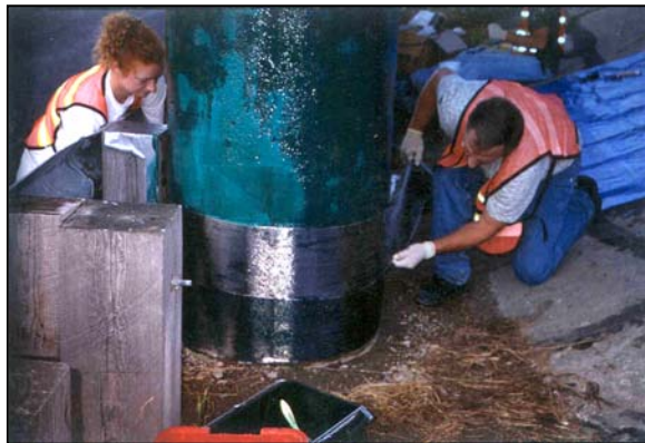
Figure A.24 Installing the fiber wrap on a column begins from the bottom.
