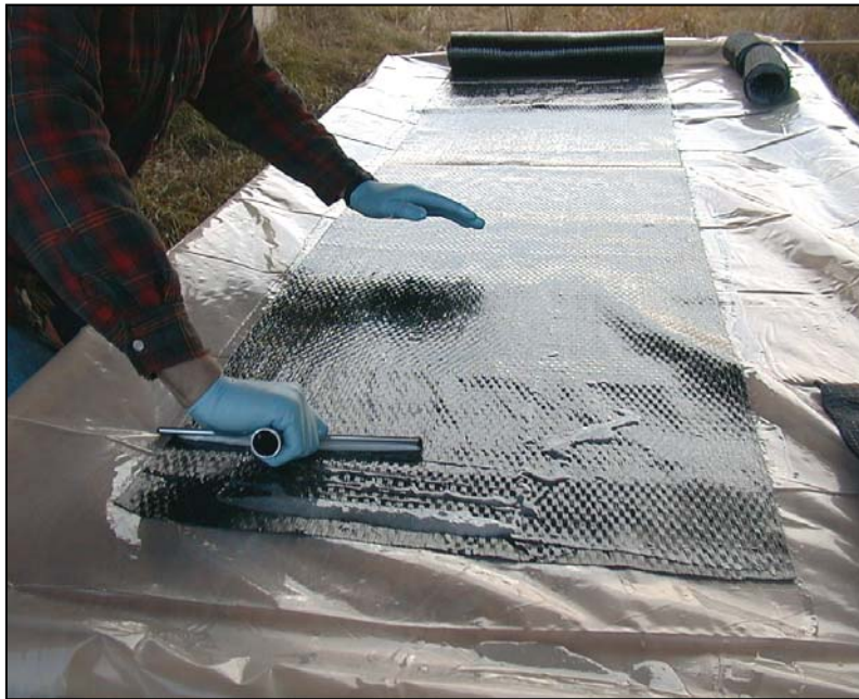
Figure A.28 Move squeegee in the direction of the fibers to work in the epoxy.
