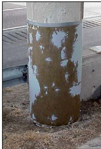
Figure A.17 Column with both the primer and putty system installed.
