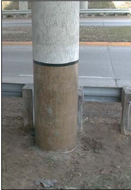
Figure A.23 Complete installation of undercoat.
