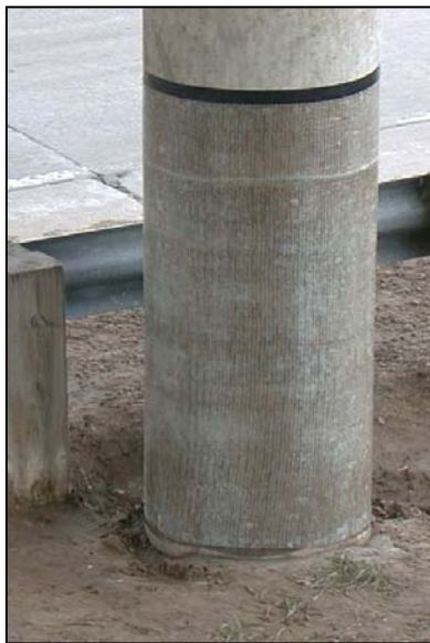
Figure 3.29 Completed glass FRP wrap at TS1.
