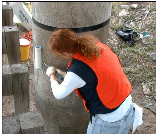
Figure A.22 Use a 3/8 in. nap roller to apply the undercoat in smooth even strokes.
