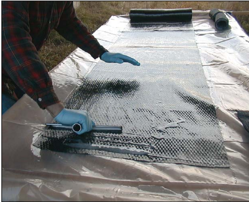
Figure 3.27 Work the epoxy into the fibers with a squeegee.
