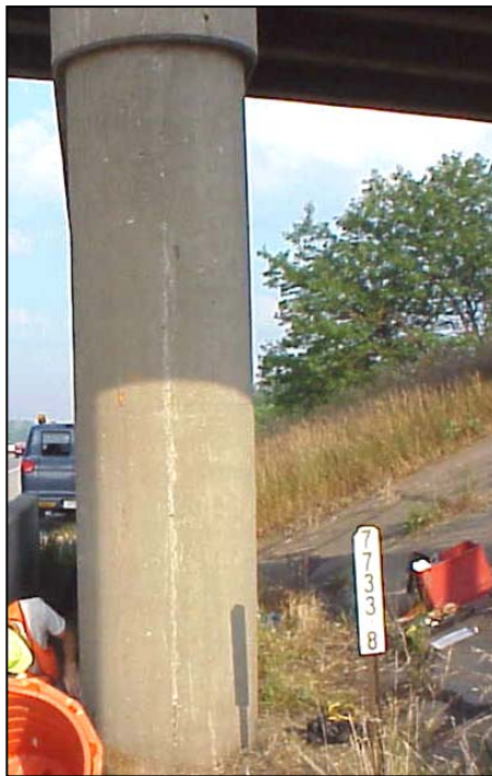
Figure 3.11 View of C5 prior to FRP wrap installation.
