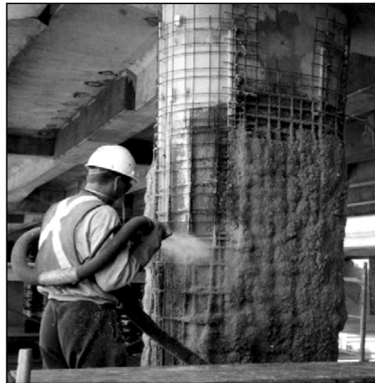
Figure 2.2 Application of an external anode with a spray-on mixture of water and cellulose fiber (11).
