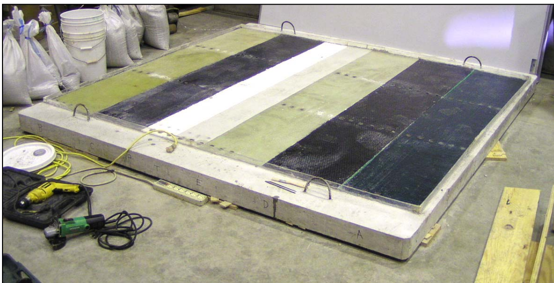
Figure 3.20 Slab 1 after all five FRP overlays and topcoats have been installed.
