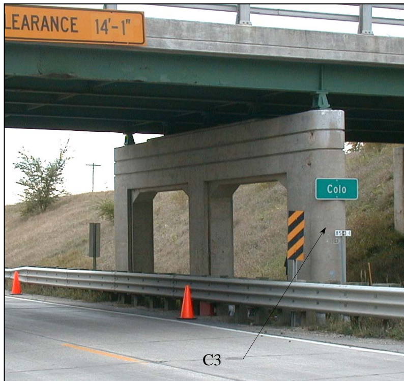
Figure 3.7 View of C3 prior to FRP wrap installation.
