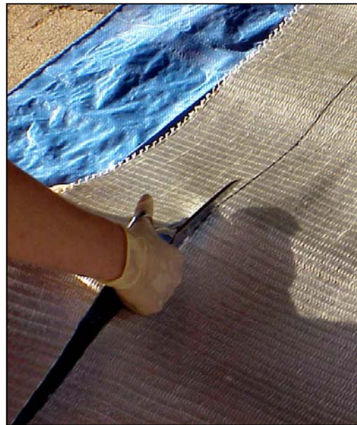
Figure 3.26 Cutting the fiber sheets.
