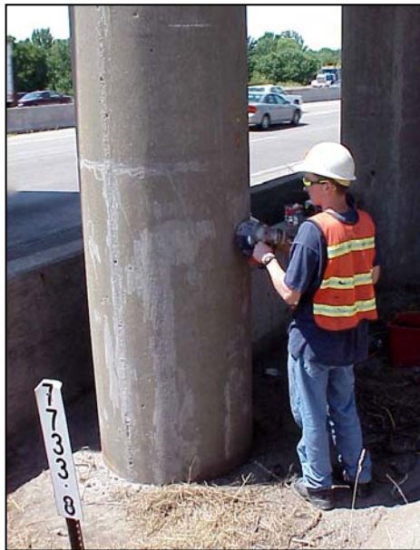
Figure 3.25 Preparation of the concrete surface.
