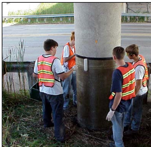
Figure A.31 Apply the overcoat with 3/8 in. nap roller in the direction of the fibers.
