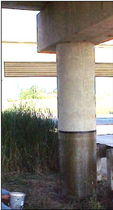
Figure A.33 Completed glass fiber wrap.
