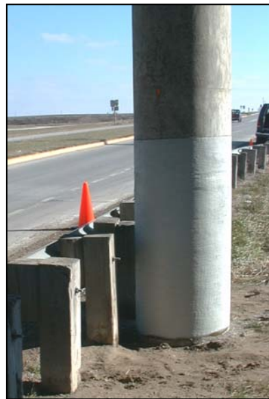
Figure 3.30 Finished FRP wrap with topcoat installed at TS1.
