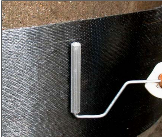
Figure A.30 Paddle wheel with a metal spline.
