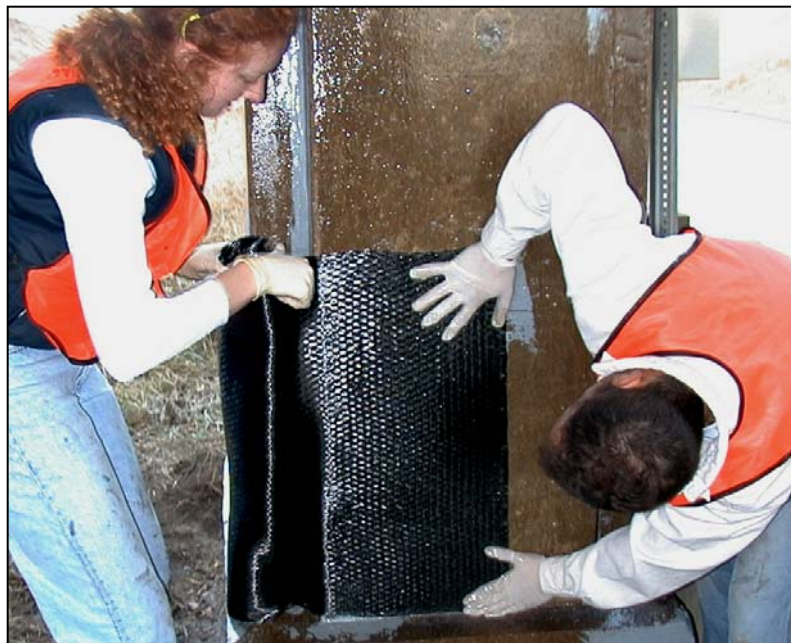
Figure 3.28 For ease in installation, unroll the FRP sheets onto the column.
