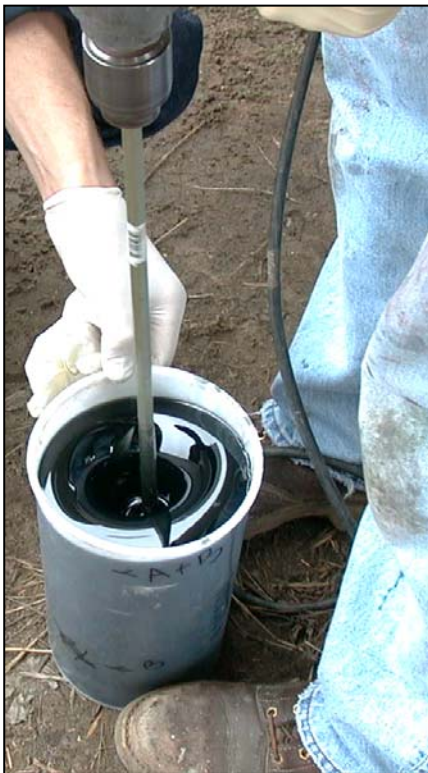
Figure A.21 Mix the epoxy's main agent and hardener in a clean container for the time specified by the manufacturer.
