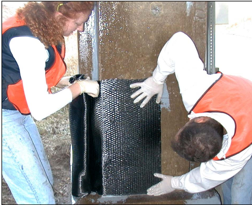
Figure A.29 Utilize two people to unroll the FRP sheet.
