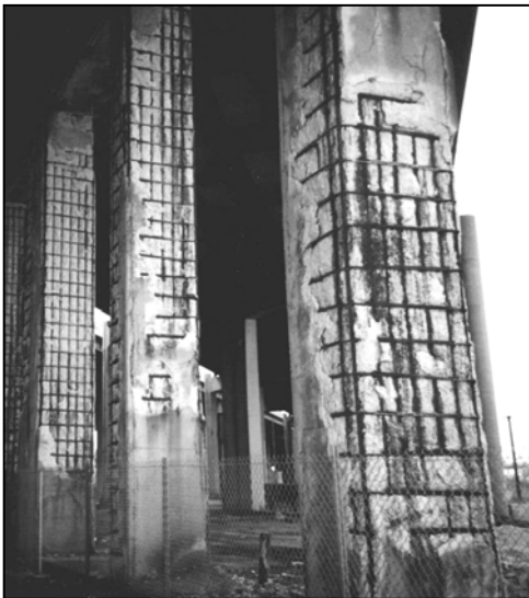
Figure 2.1 An extreme example of spalling concrete (11).
