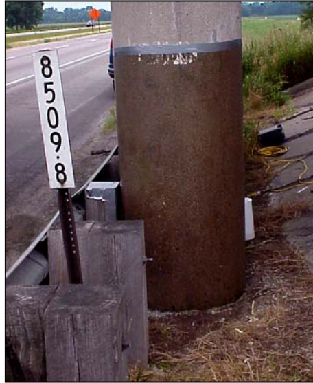
Figure A.14 Column with primer system installed.
