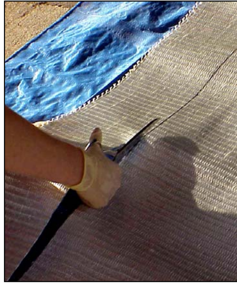
Figure A.19 Use scissors or a rotary knife to cut the E-glass sheets.
