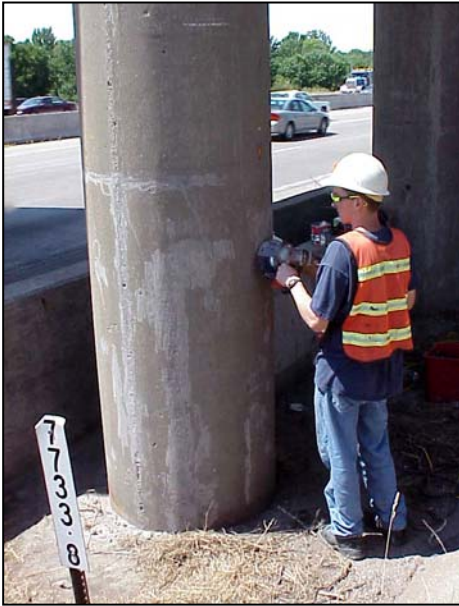
Figure A.11 Grind the concrete surface to remove any unevenness.
