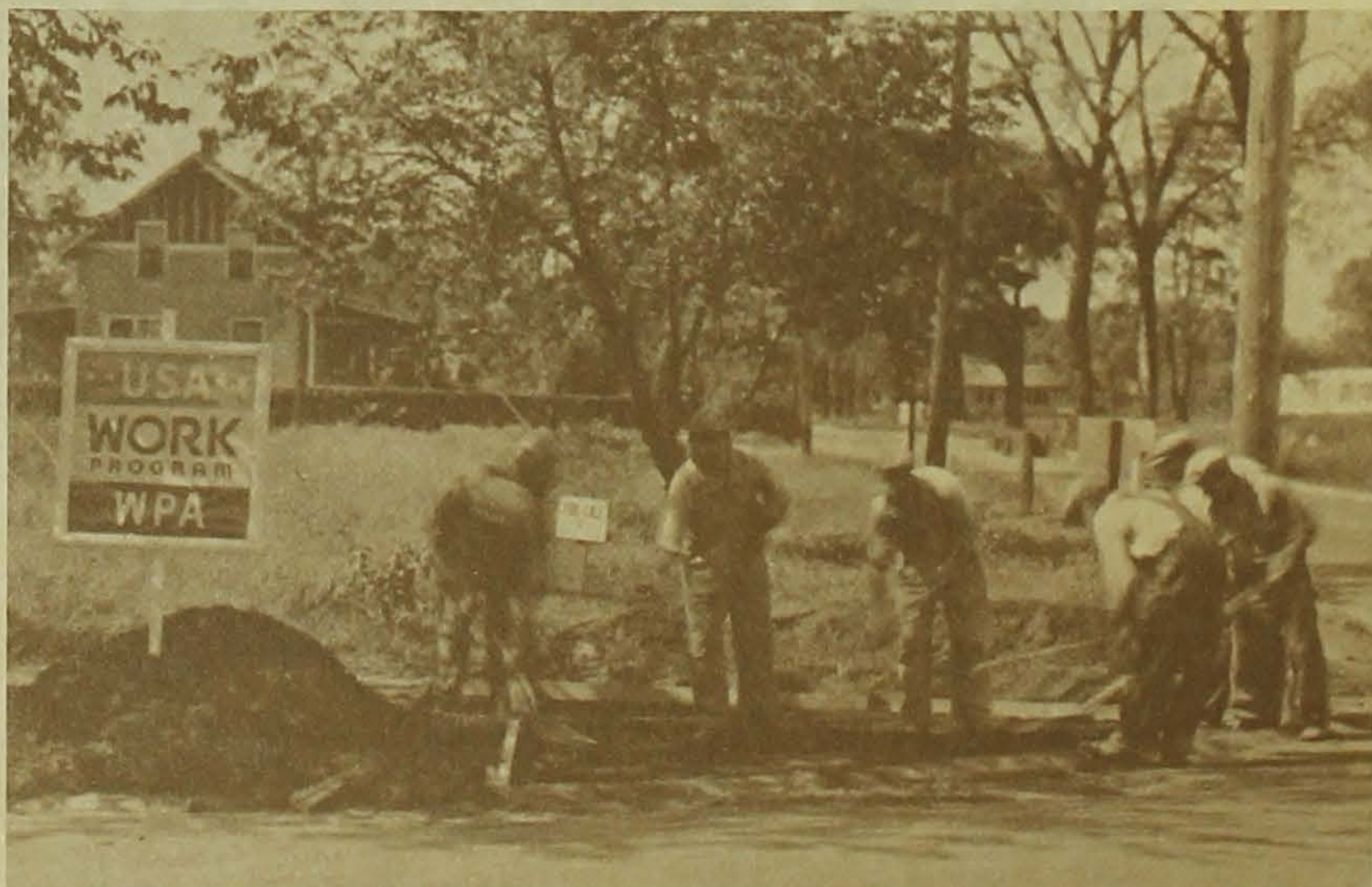
A WPA sidewalk repair project at Waterloo.
