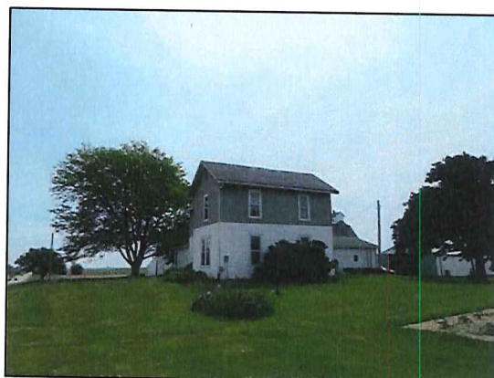
PHOTO 6: NORTH AND WEST ELEVATIONS
