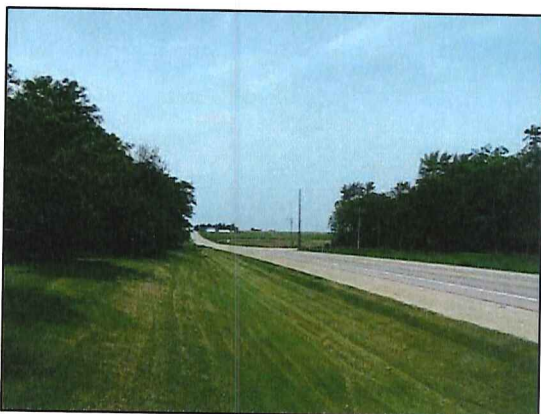
PHOTO 2: VIEW WEST OF SUBJECT ON HIGHWAY 30
