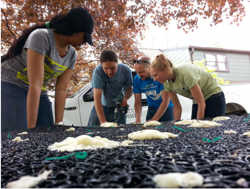
This view shows the people attaching the steel frame for the lighted sculpture to the VFI. Small, individual pours of marine foam (the white substance in this photo) was used to hold the 3 layers of biofilter material together.
