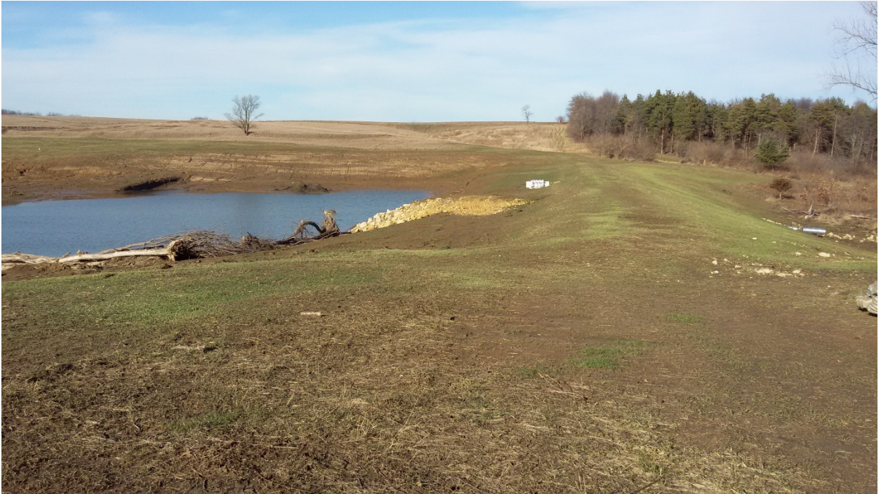
West Pond Shortly After Construction (partially filled)
