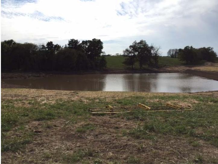
Left: this grade stabilization structure was completed late September 2015. Seeding and mulching of the disturbed area is shown. This structure quickly filled as the drainage area is 157 acres. This is a DNR permitted site.
