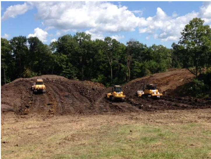
Left: Dozers work to construct a grade stabilization structure. This structure was completed September 2015 and has a drainage area of 86 acres.
