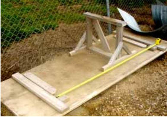
c. Jig for assembling individual components
