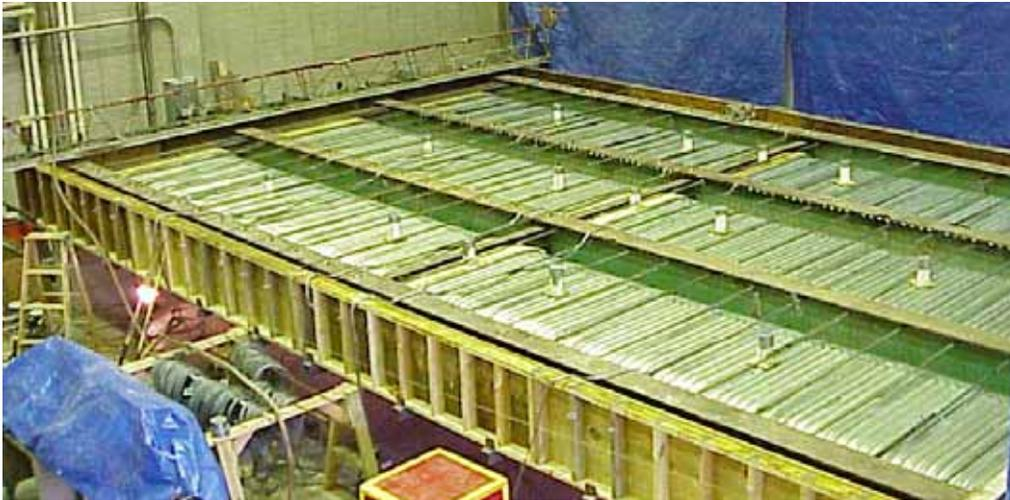
b. Formwork and reinforcement in the model bridge
