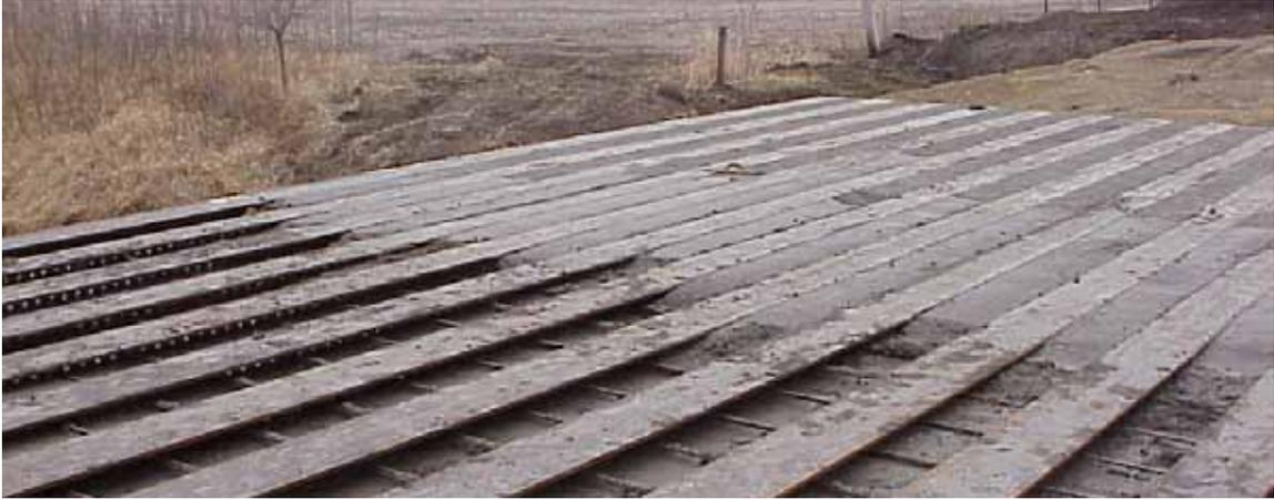
a. Concrete struck off even with the top flange
