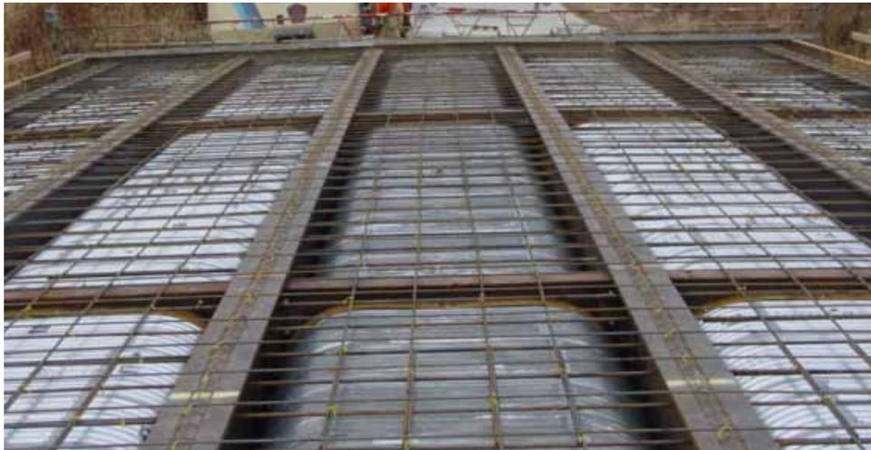
Figure 4.13. ASC and crack control reinforcement prior to concrete placement.
