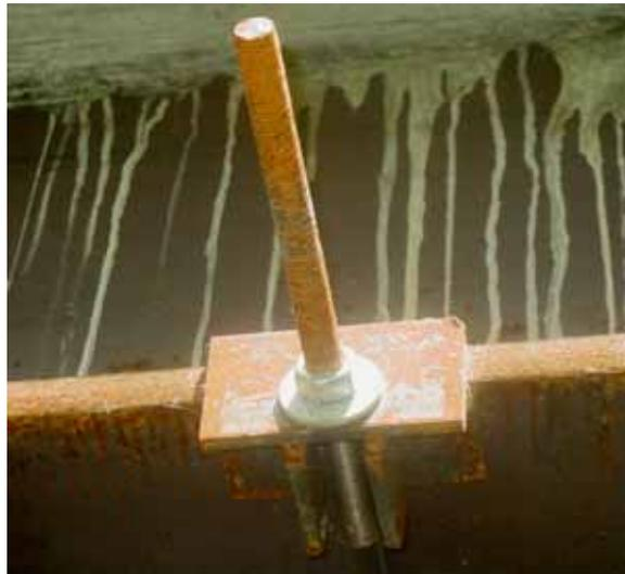
b. Installed tension clip
