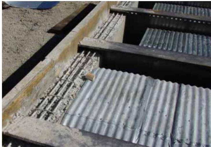
b. Custom rolled arched formwork abutted to the backwall
