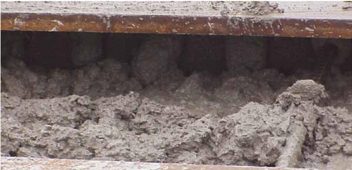
b. Concrete flowing through the ASC holes forming shear dowels
