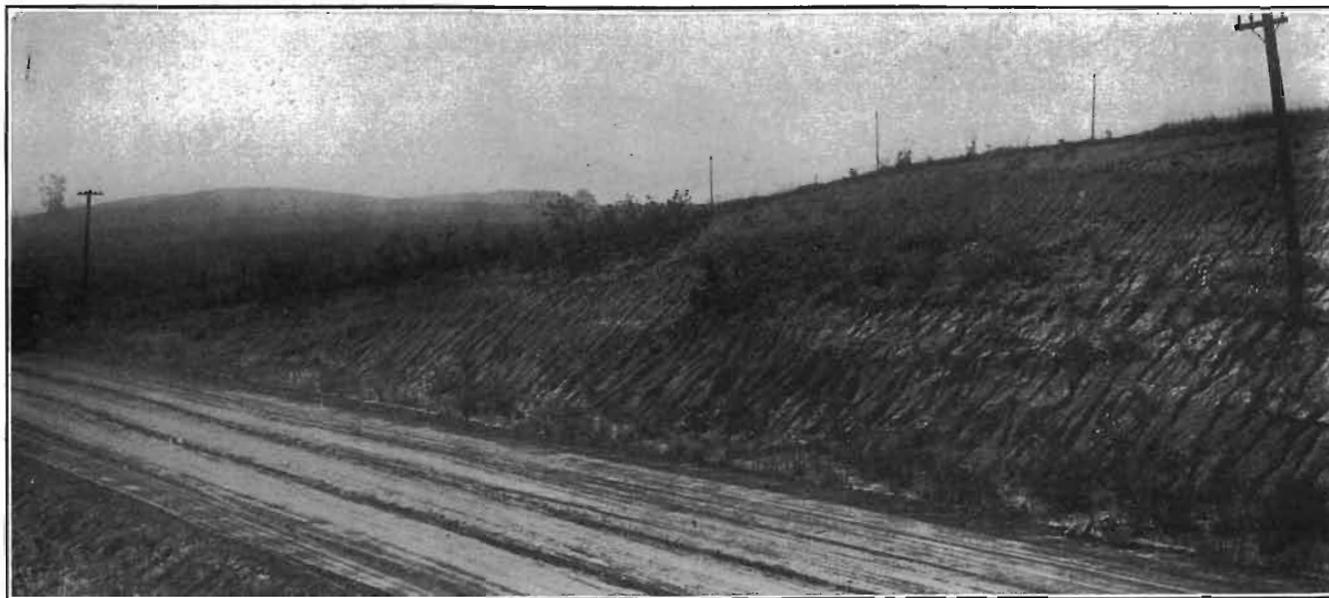
FIG. 53.—Cut in Windsor township, Fayette county, showing Iowan till over loess on Kansan gumbootil.
