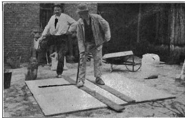
FIG. 82.—Tamping the hydraulic gypsum floor.
