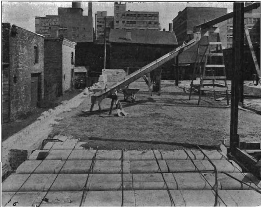
FIG. 76.—Gypsum floor tile showing conduits, and surfacing of same with concrete. Castle Hotel, Omaha. Courtesy V. G. Marani.
