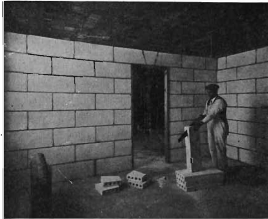
FIG. 64.—Sawing a four inch block for furring. Courtesy Beaver Board Co.
