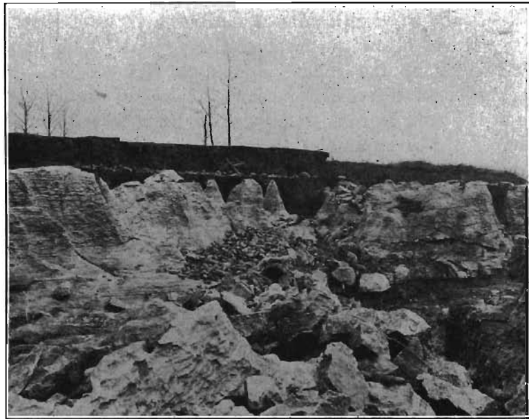
FIG. 12.—Gypsum at the Vincent Clay pit, exposed by hydraulic stripping, described somewhat fully in the text. Photo by Lees.
