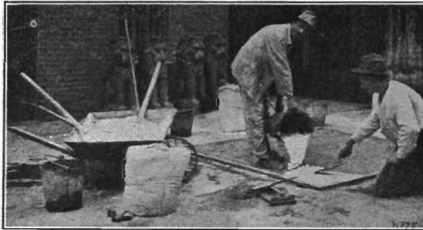
FIG. 80.—Pouring the hydraulic gypsum.
