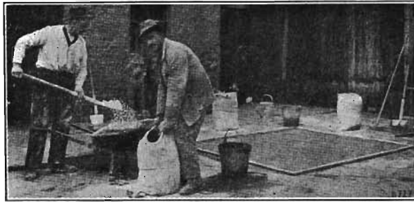
FIG. 79.—Mixing the hydraulic gypsum.
