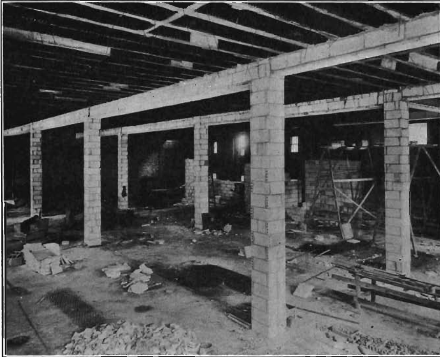
FIG. 63.—Gypsum blocks used as fireproofing. Courtesy of V. G. Marani.
