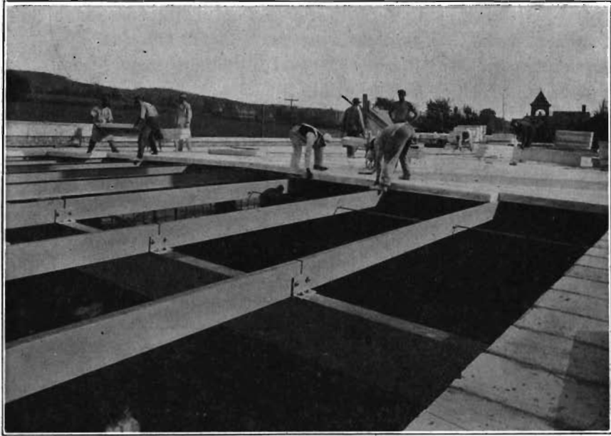
FIG. 74.—Laying precast gypsum roof tile on purlins. Courtesy United States Gypsum Co.
