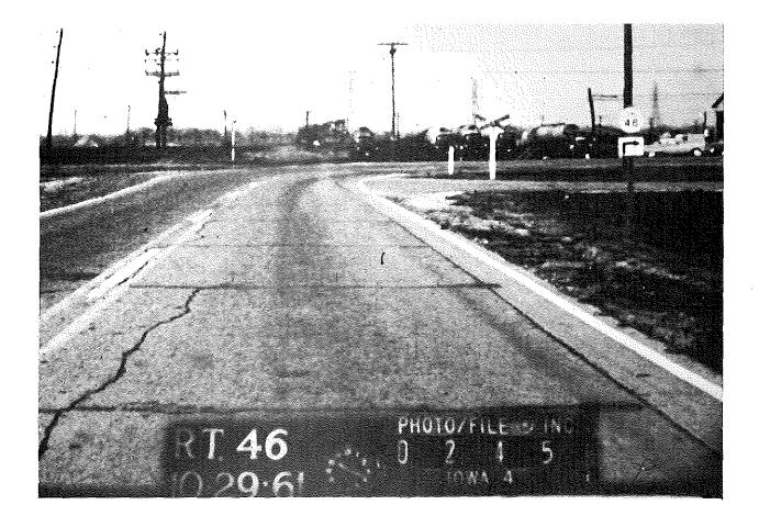
Unprotected grade crossing on primary highway. Sharp curve (15 mph advisory speed), with access on curve. Iowa 46, October 29, 1961, 10:20 A.M., 2.45 miles from control point.
