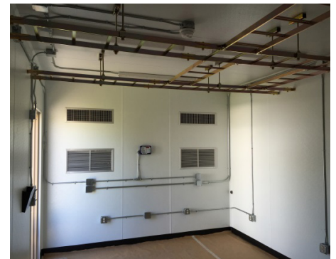
Inside the new hut structure.
