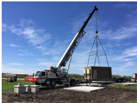
Lowering the 12 ft. by 20 ft. switching point structure on the foundation at the new location.
