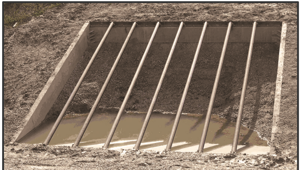
Safety treatment for cross-section drainage culverts Photo: Midwest Roadside Safety Facility (MwRSF) University of Nebraska-Lincoln
