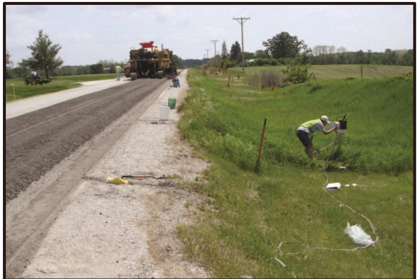
Installation of weather station
