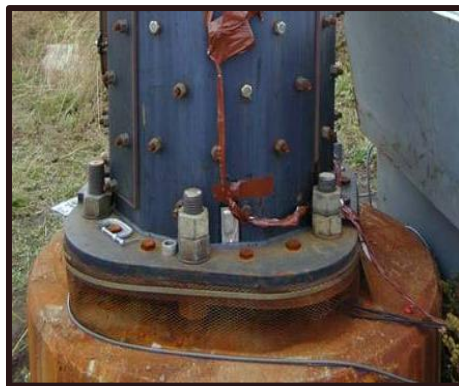
Bolted Reinforcing Jacket
