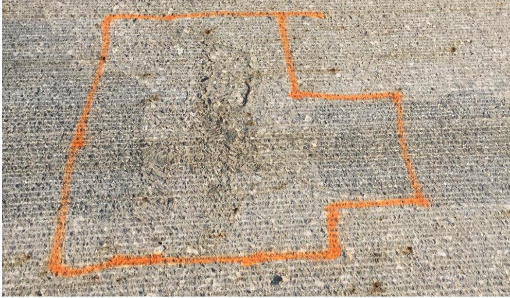
Figure 3. Area marked for more in-depth removal
