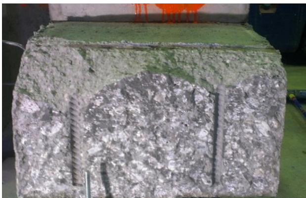
d) Bond interface (overlay concrete)
