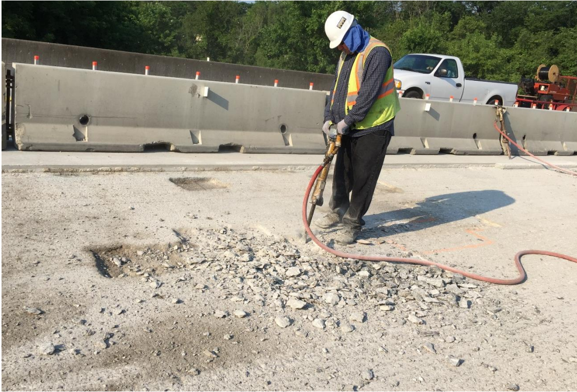
Figure 4. Removal of unsound concrete using jackhammer
