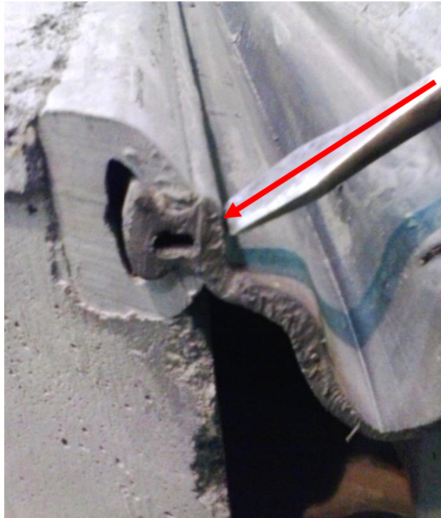
Figure 18. D.S. Brown strip seal
