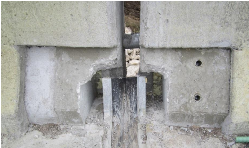
Figure 5. Field construction of termination detail
