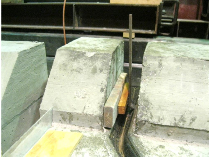
Figure 52. Wood blocking used between mid-height barrier rails with Watson Bowman Acme gland installation tool
