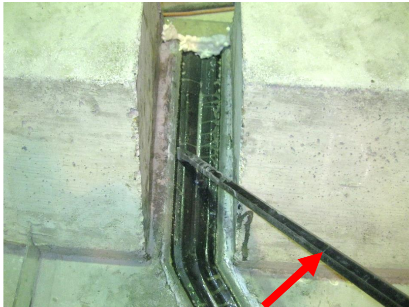
Figure 53. Use of a crowbar to install D.S. Brown gland
