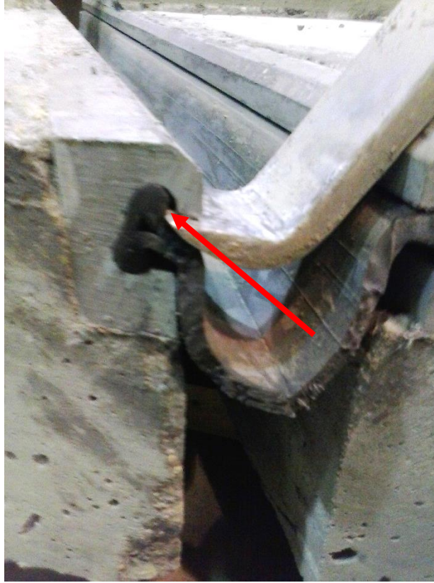
Figure 20. Watson Bowman Acme strip seal
