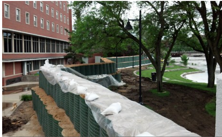
Flood barriers erected at the Memorial Union on the University of Iowa campus in May 2013.
