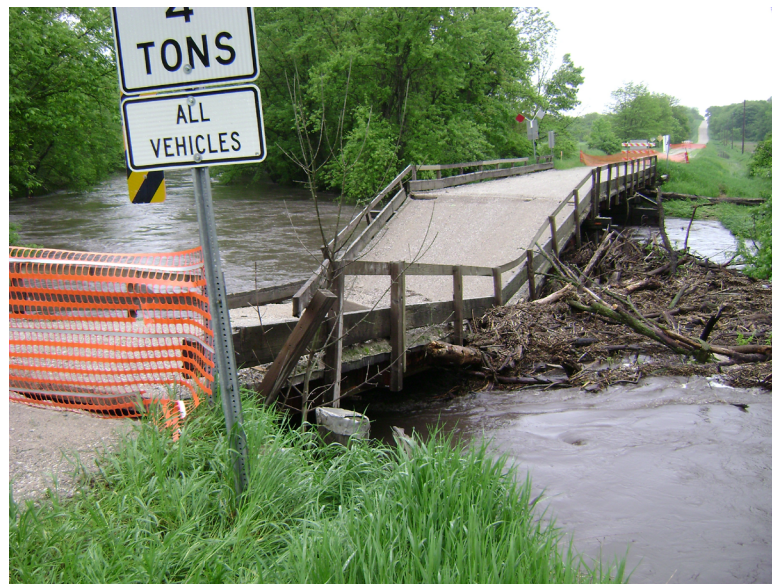
Damage to a bridge in rural Story County during the May-June 2013 flooding.
