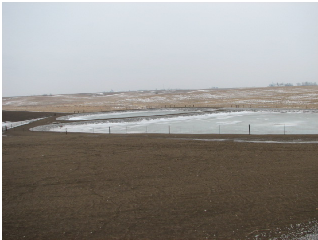
Lagoon 1 – 2.08 ac. 2.51 million gal. 121 days storage Lagoon 2 – 1.0 ac. 1.24 million gal. 60 days storage. Total Storage 181 days.
