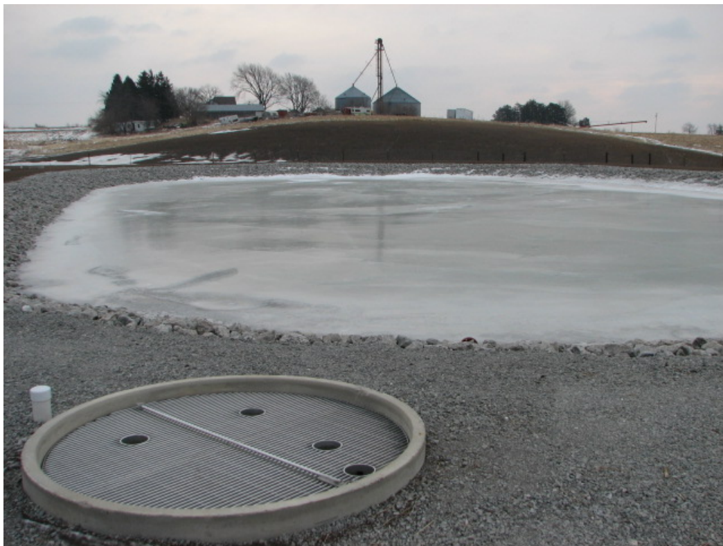
Lagoon #2 and Controlled Discharge Outlet intake.
