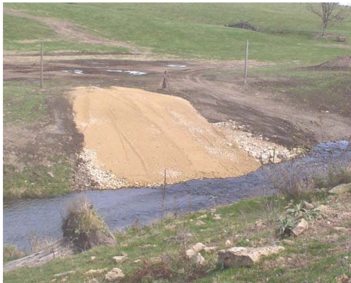
The picture shows one of three cattle approaches near completion on the Kremer farm. Exclusion fencing was installed on the sides of the approach and along the stream.
