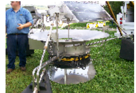
Lake Circulators Final Inspection
