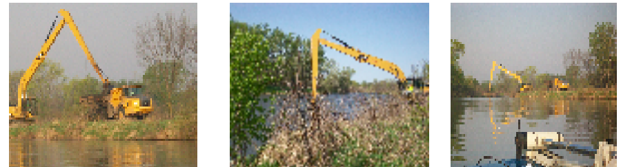
West End/North Shore Excavation – April/May, 2010 @ ~6,174 CY
