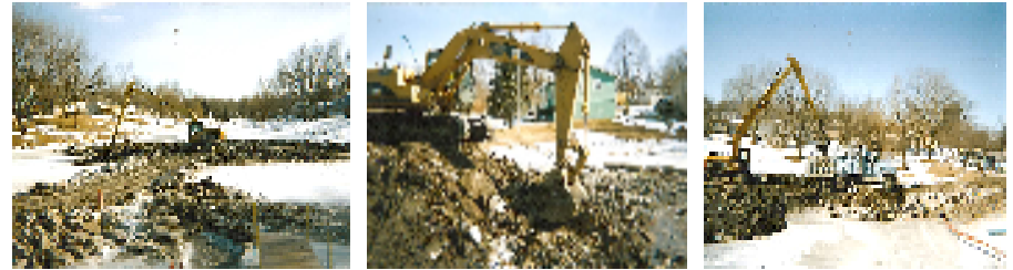
Finger Pond Excavation – February, 2009 @ ~1,300 CY
