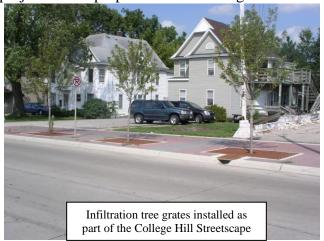
paving on the sidewalks serves as a walking space, but is also essential to stormwater management as special grading was installed to ensure it's proper drainage into the installed BMP's. Contributions from the WIRB grant to this project totaled \$8,400.
