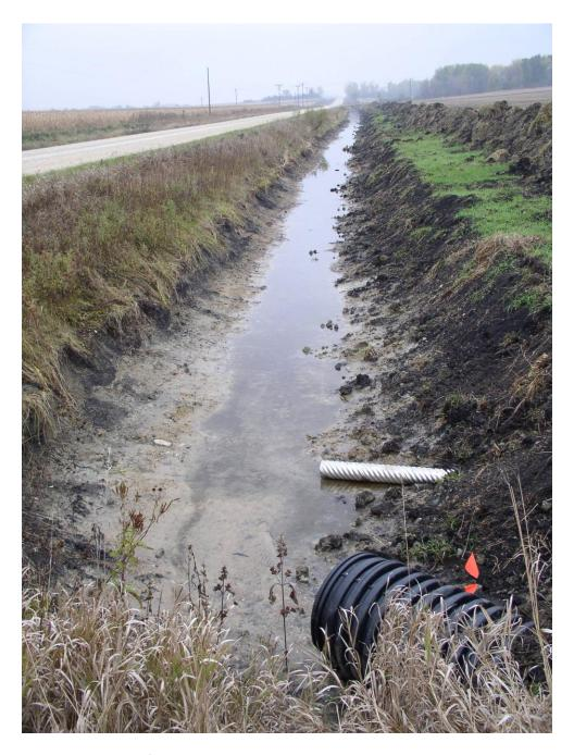
Shown here is the large outlet for the project. As can be seen on the cleaned out road ditch, the grade is extremely flat. It was loaded with wetland vegetation before the cleanout and those plants will quickly reestablish in the new wider bottom. This will allow for some nutrient and pesticide reduction of the tile water as it heads downstream.
