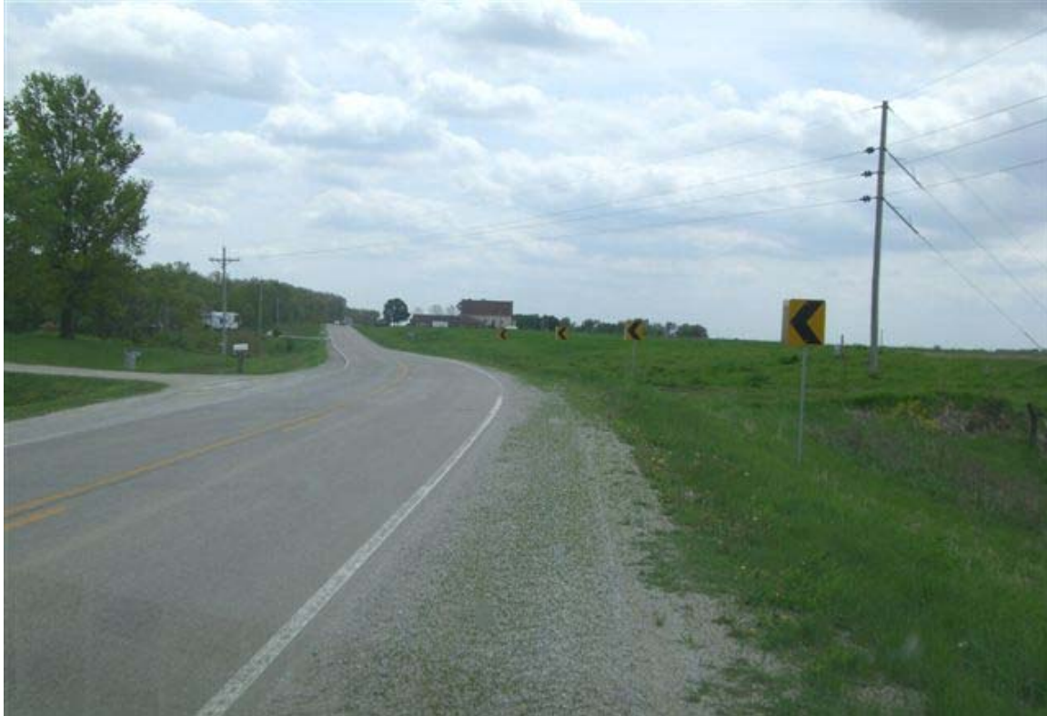
Figure C.4. Existing signing and pavement markings
