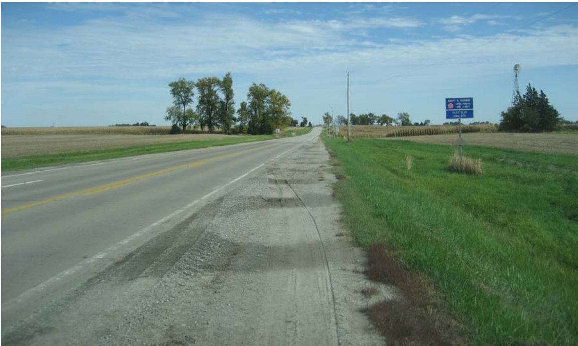
Figure D.4. Shoulder conditions with worn edge line
