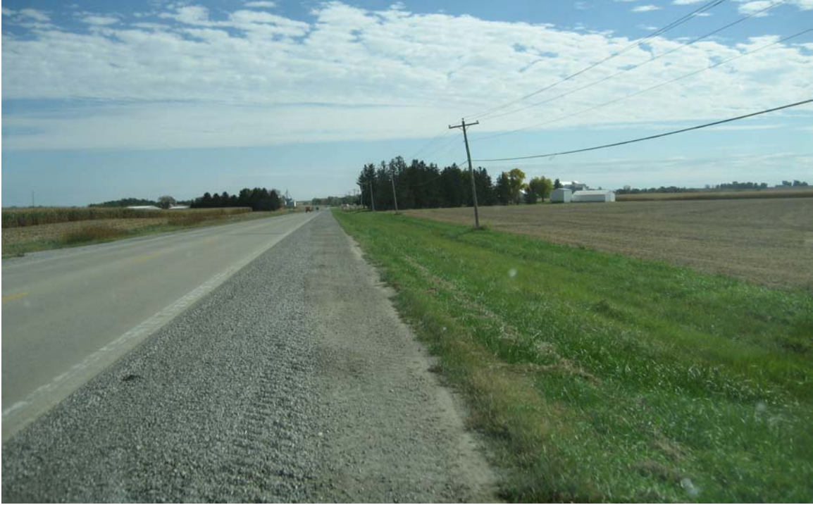
Figure D.3. Wide granular shoulder with worn edge line
