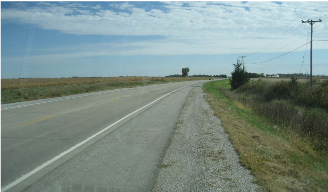
Figure D.2. Partially paved shoulder
