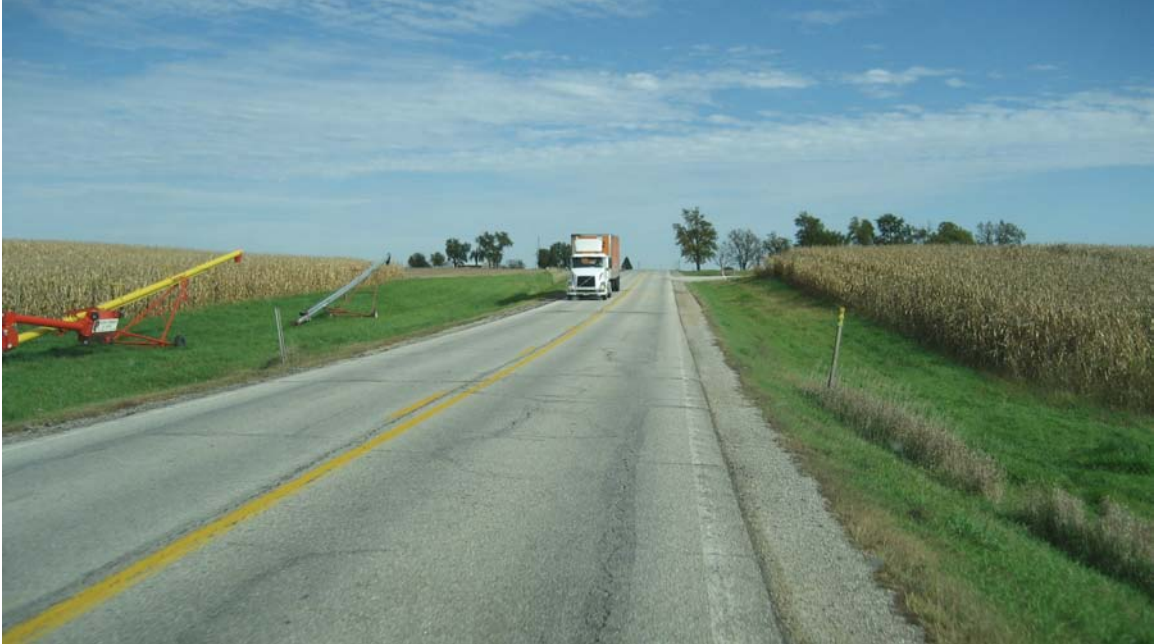
Figure D.5. Narrow granular shoulders and right of way with worn edge line
