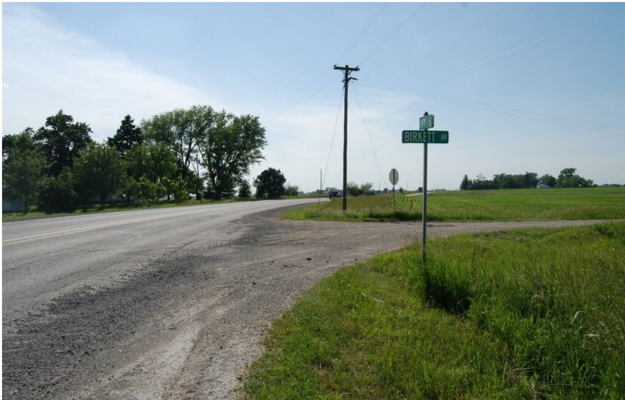
Figure D.32. Burkitt Avenue intersection with US 6, utility pole with downguy in clear zone
