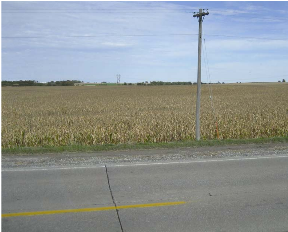
Figure D.9. Utility pole with downguy in clear zone
