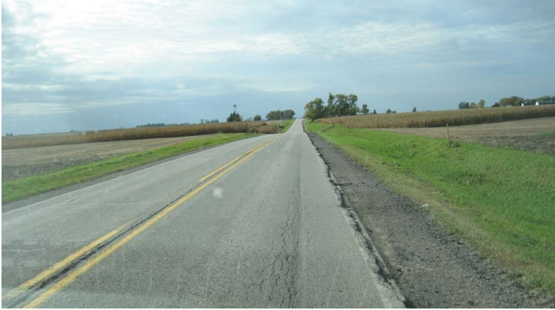
Figure D.11. Pavement edge conditions
