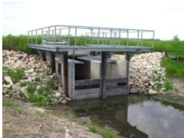
Pickerel Lake in drawdown condition (left). The outlet structure replaced at Pickerel Lake now incorporates both the ability to control water levels and a fish barrier to keep rough fish out of the lake.
