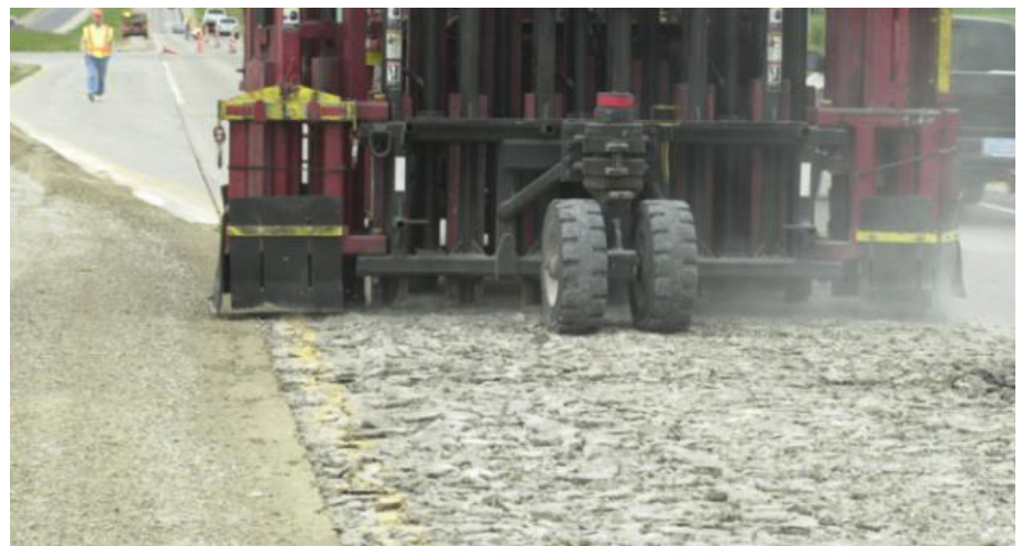
Rubblization using a multiple-head breaker
