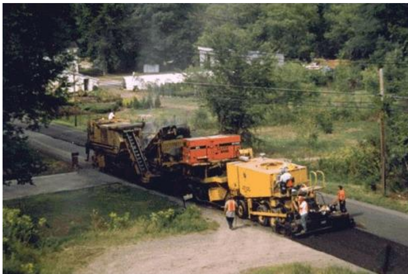
Figure 9. Cold in-place recycling
