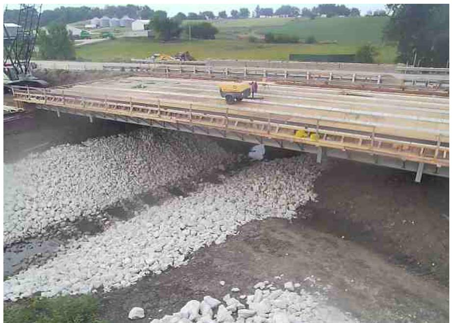
*Slide-in bridge during accelerated bridge construction next to the original IA 92 Massena Bridge*
