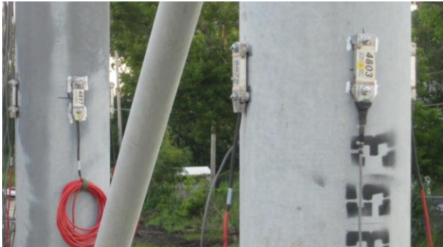
View of a strain gage attached on a truss member
