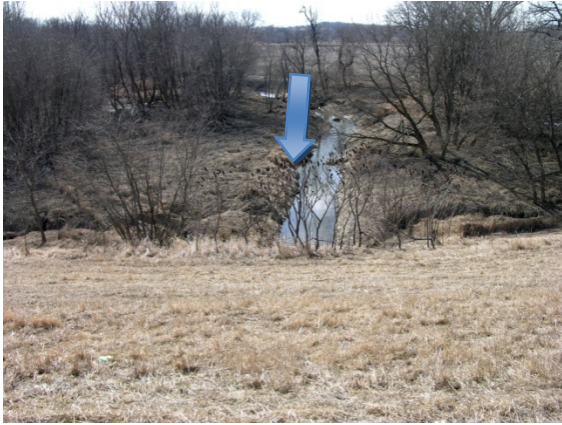
The stream is well aligned with the culvert axis. Steep slopes from all the culvert sides cut strong ditches merging upstream the culvert.
