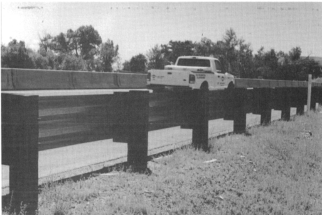
Figure 8.21. Wood post thrie-beam barrier (AASHTO 2002).
