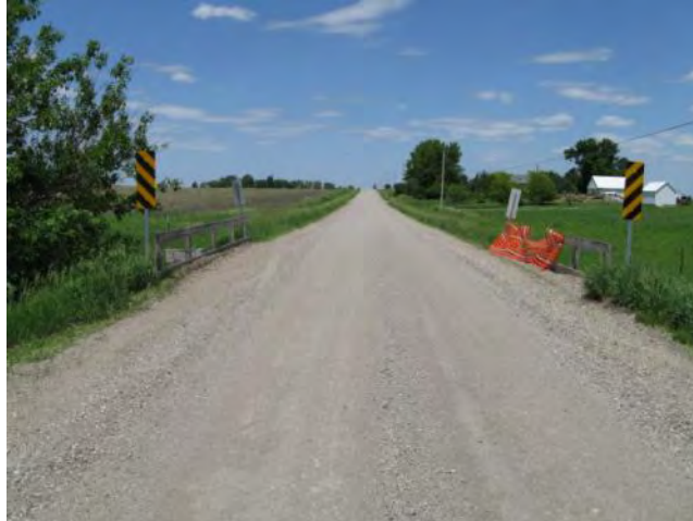
Figure 4.3. LVR timber bridge, with damaged bridge rail, included in the state inventory
