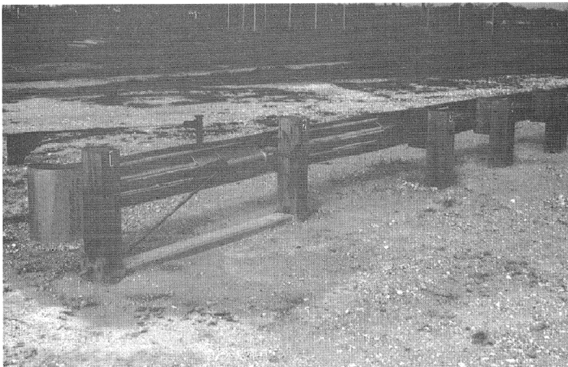
Figure 8.5. Slotted rail terminal (SRT-350) with 1.2 m [4 ft] flare (AASHTO 2002).
