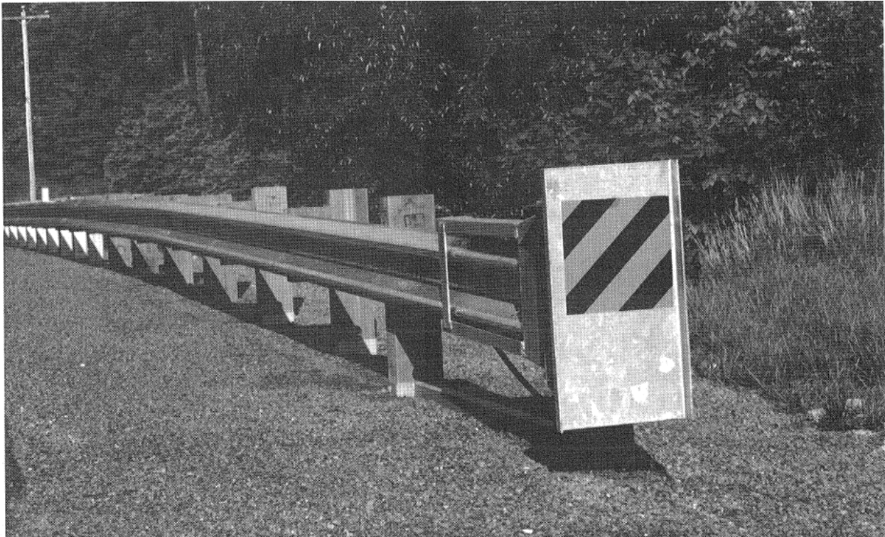
Figure 8.10. Extruder Terminal (ET-2000) (AASHTO 2002).
