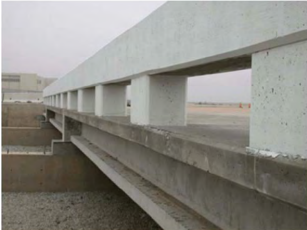
Figure 8.30. Layout for open concrete bridge rail attached to inverted tee bridge deck system (Faller et al. 2004).
