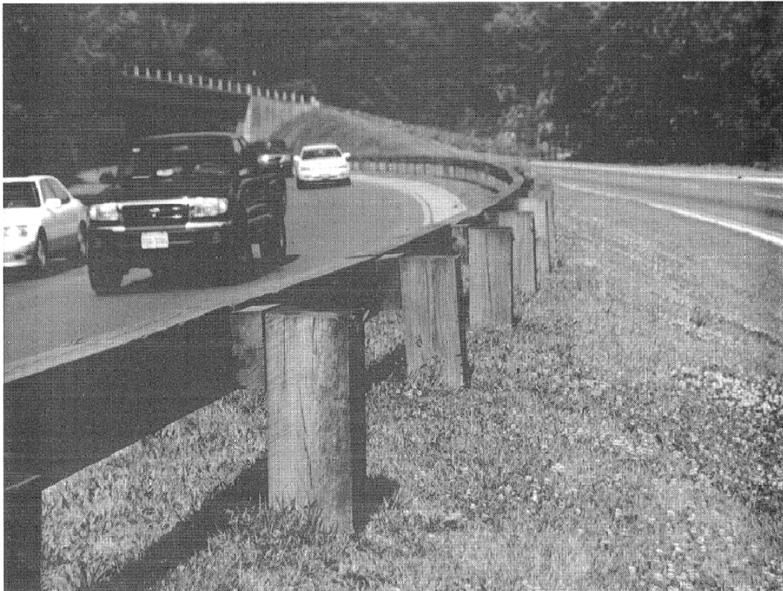
Figure 8.23. Steel-backed timber guardrail (AASHTO 2002).
