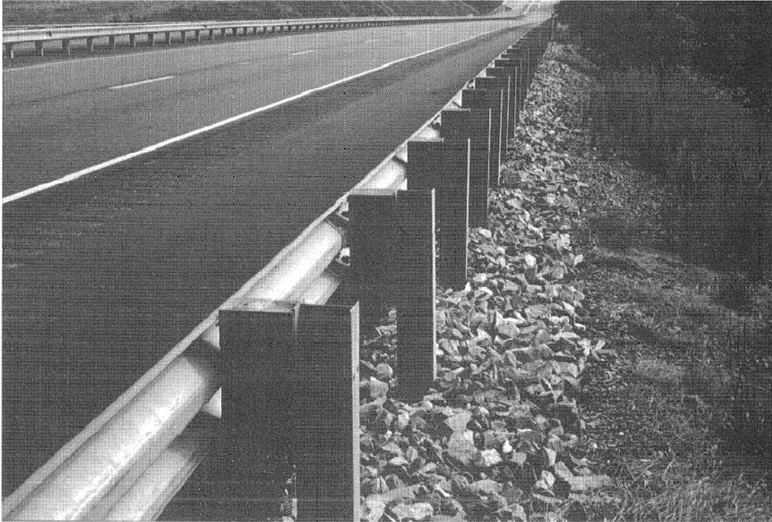
Figure 8.19. Steel post W-beam with wood block-outs (AASHTO 2002).
