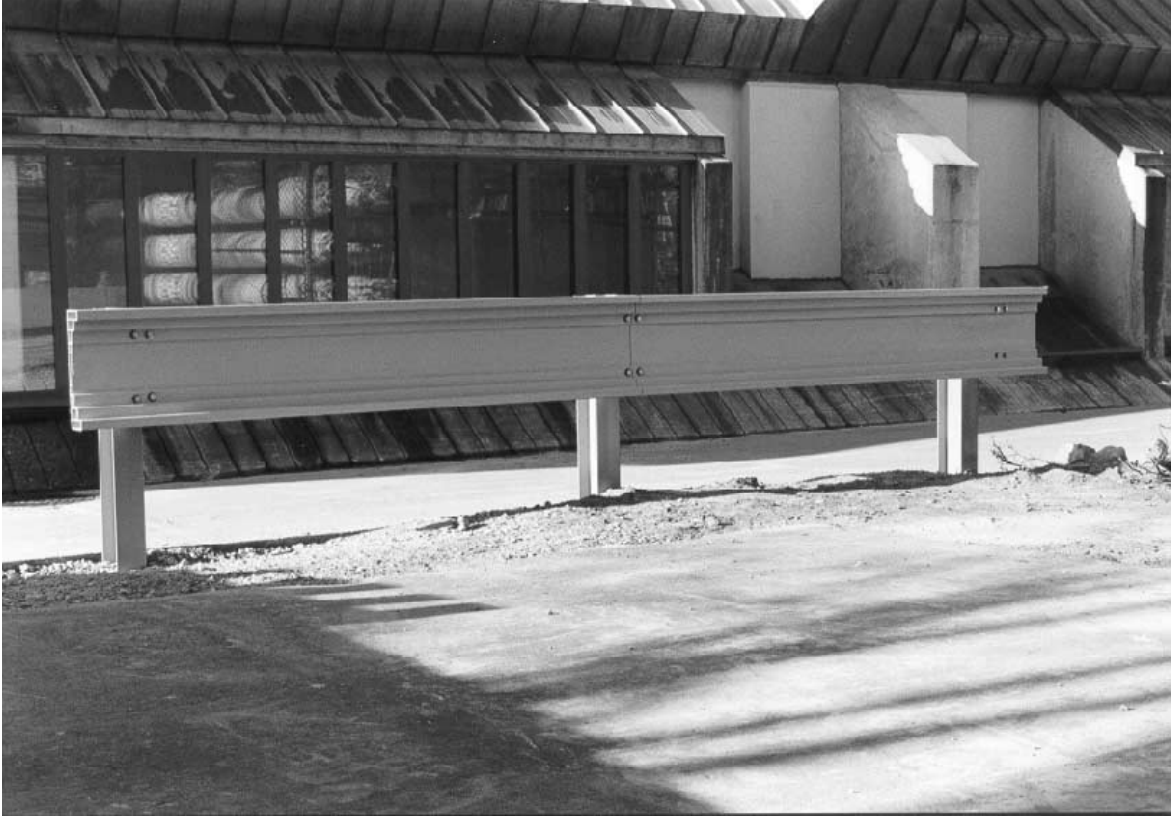
Figure 8.25. Demonstration installation of the composite guardrail (Bank et al. 2001).
