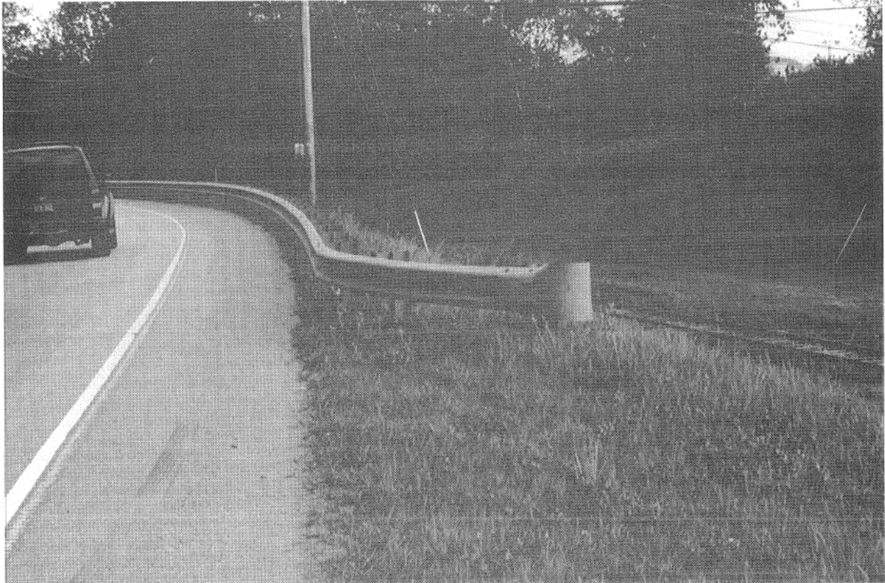
Figure 8.7. Vermont low-speed, W-beam guardrail end terminal (AASHTO 2002).
