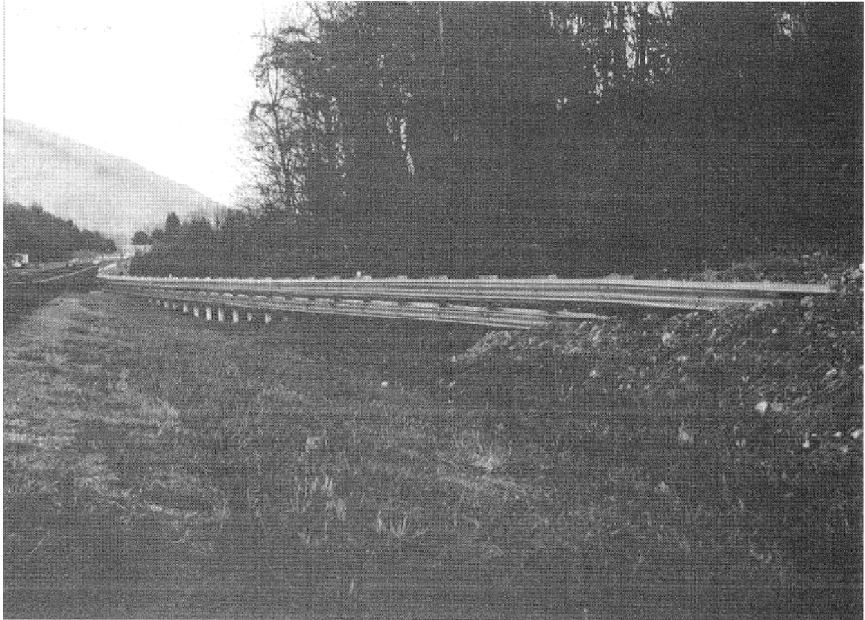
Figure 8.3. W-beam guardrail anchored in backslope (AASHTO 2002).
