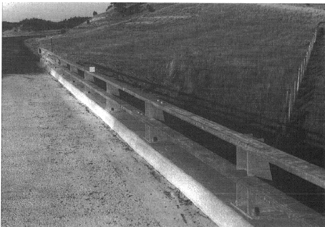
Figure 8.28. Wyoming two-tube bridge railing (AASHTO 2002).
