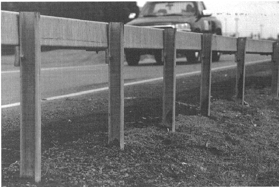
Figure 8.18. Weak post box beam barrier (AASHTO 2002).
