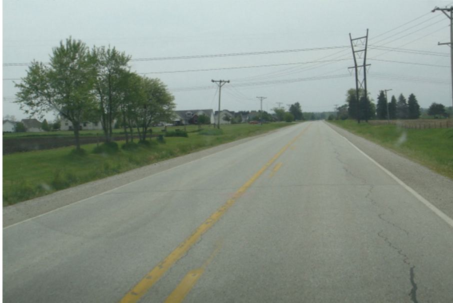
(a) Longitudinal crack
