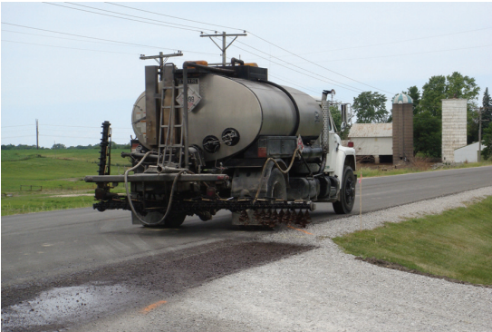
(b) Tack coating process
