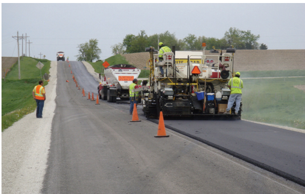
(c) Intermediate HMA overlay process
