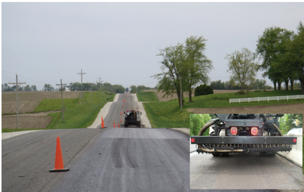
(b) Tack coating process
