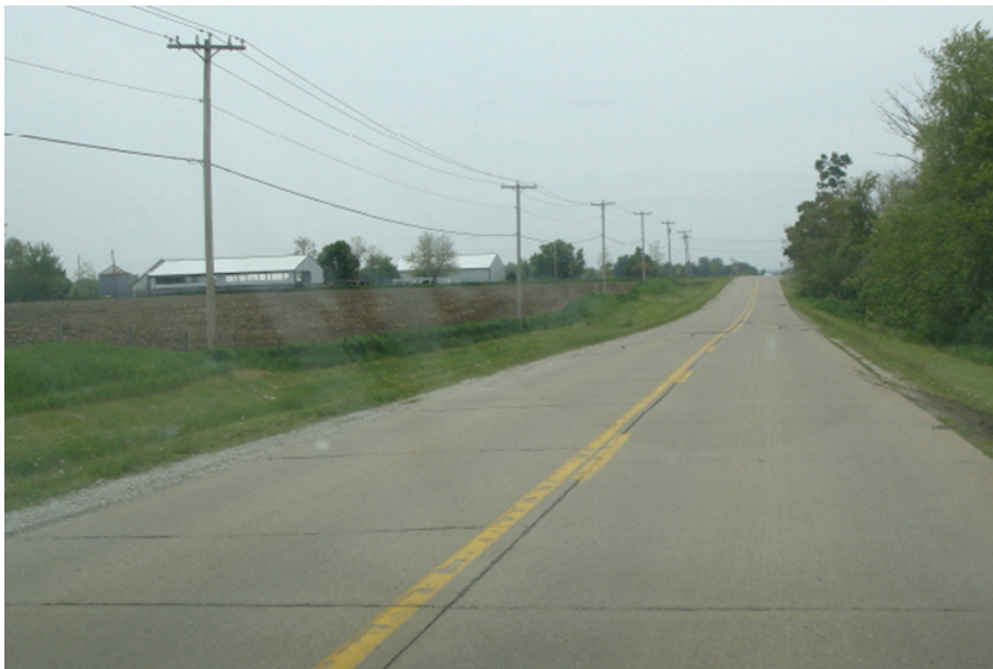
(b) Transverse cracks
