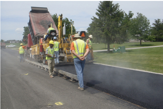
(c) Intermediate HMA overlay process
