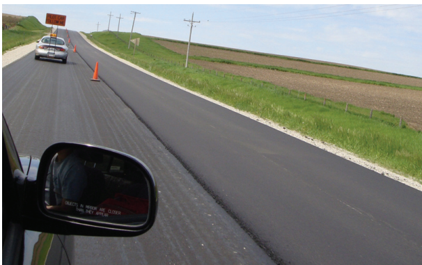
Figure 5-4. Pictures of CIR-foam, tack coating, and HMA overlay processes
