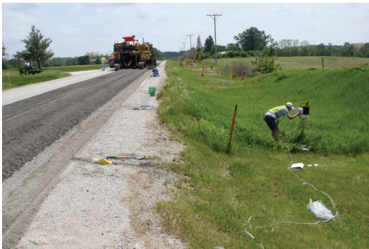
(c) Installation of weather station
