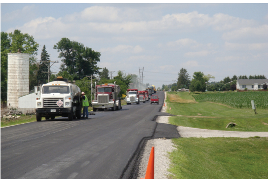
Figure 6-3. Pictures of CIR-CSS-1-emulsion, tack coating, and HMA overlay processes
