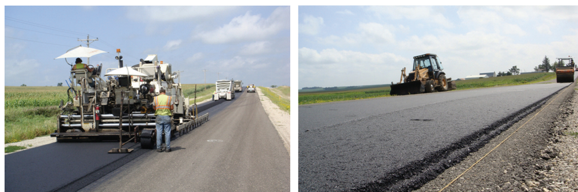
(c) Intermediate HMA overlay process
