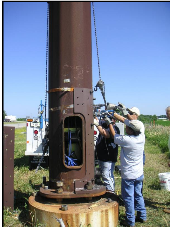
Figure 1.1 – Installation of the reinforcing jacket
