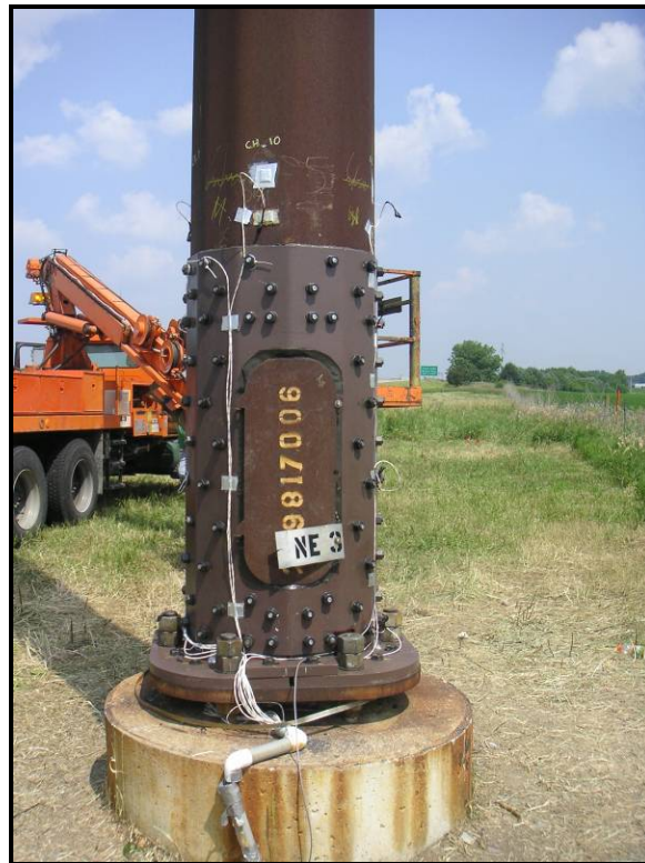
Figure 2.6 – Base of high-mast tower after installation of reinforcing jacket and all instrumentation
