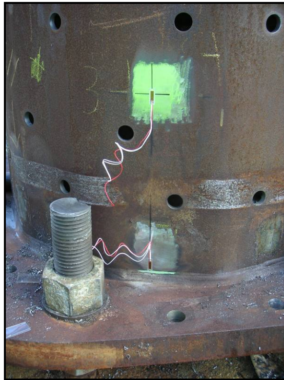
Figure 2.4 – Strain gages installed on the existing high-mast tower at the toe of the base weld and 12 in. above the base plate
