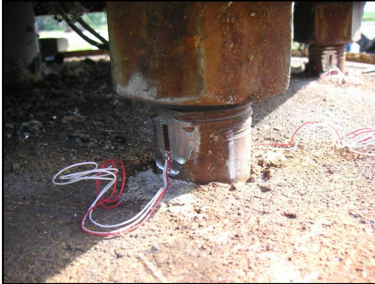
Figure 2.5 – Strain gage installed on the anchor rod between the concrete foundation and lower leveling nut
