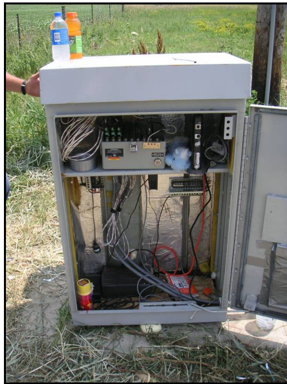
Figure 2.1 – Weather-tight enclosure adjacent to the high-mast tower used to house the data acquisition and communications equipment
