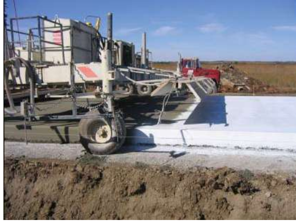
Figure 6. Uniform application of curing compound to slab surface and sides (Taylor et al. 2006)
