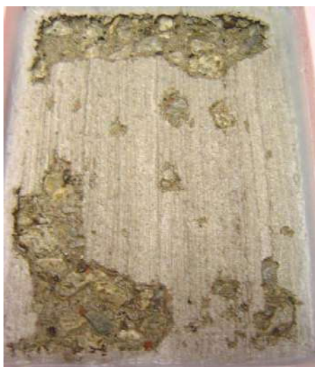
Figure 2. Concrete scaling caused by deicing chemicals (Sutter 2008)
