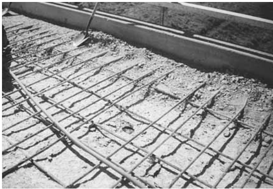
The Quasqueton bridge after removal of unsound concrete. Note that both top and bottom steel are visible in some areas and there is at least one hole clear through the deck.
