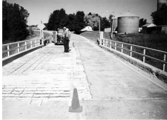
The Quasqueton bridge after removal of unsound concrete. Note that both top and bottom steel are visible in some areas and there is at least one hole clear through the deck.
