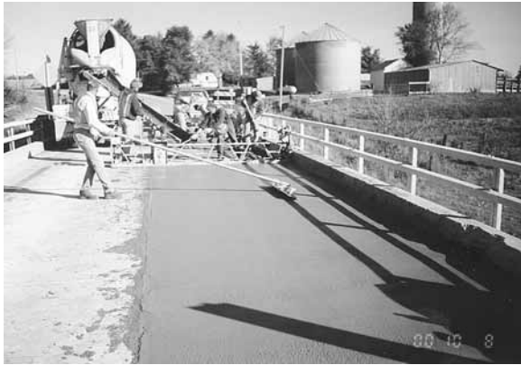
PCC placement on the Quasqueton bridge
