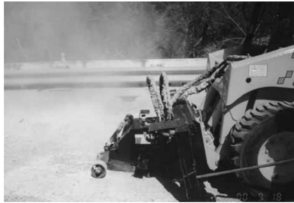
Use of milling, high-pressure air blast and jack hammers to remove deteriorated concrete from the bridge decks.
