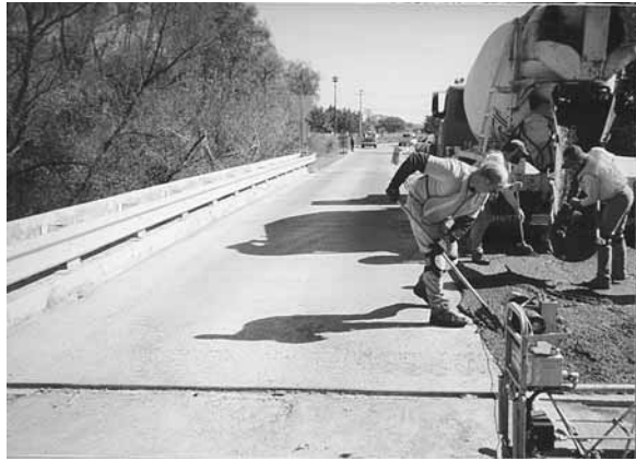
PCC Placement on the Independence Bridge. East-bound lane of the Independence bridge, showing the wheel track (arrowed) from a farm vehicle that passed over it approximately 40 minutes after PCC placement.
