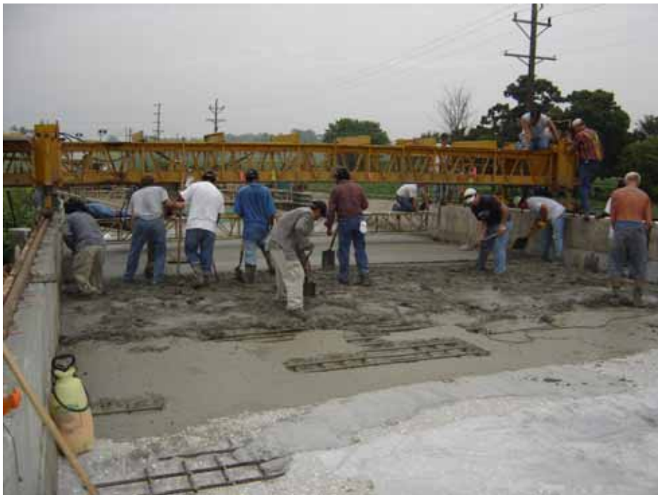
Bridge Deck overlay on IA-330 in Marshal county, summer of 2005.
