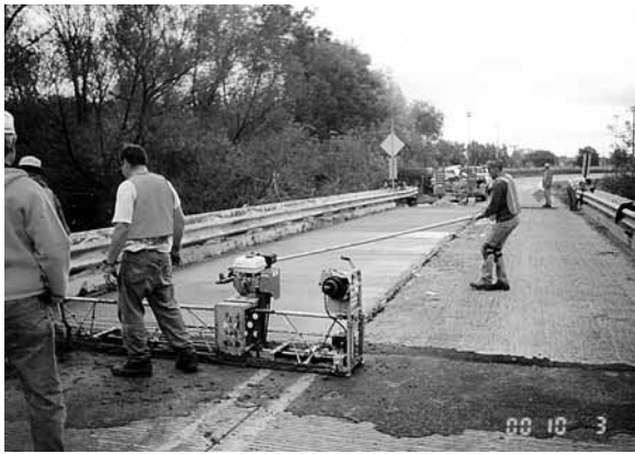
PCC Placement on the Independence Bridge. East-bound lane of the Independence bridge, showing the wheel track (arrowed) from a farm vehicle that passed over it approximately 40 minutes after PCC placement.
