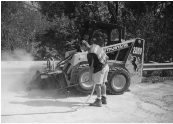
Use of milling, high-pressure air blast and jack hammers to remove deteriorated concrete from the bridge decks.
