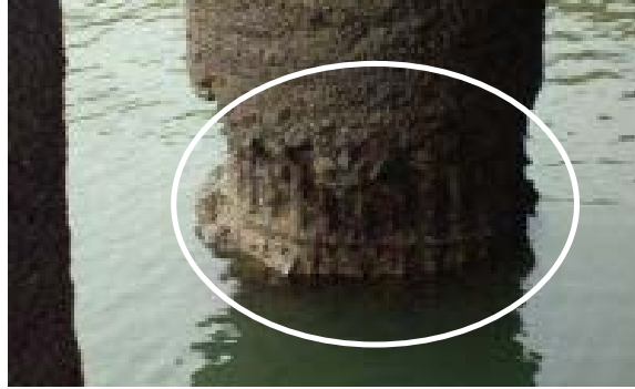
Figure 1.4. Prestressed concrete marine pile with spalling and reinforcement corrosion in a marine environment (Port Strategy 2007)
