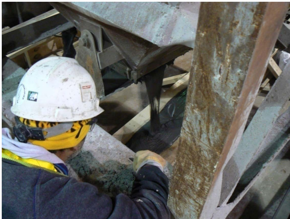
Figure 4.18. Beginning of first pour of UHPC units
