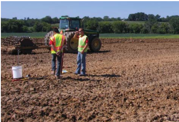
Compaction and testing of unsuitable fill
