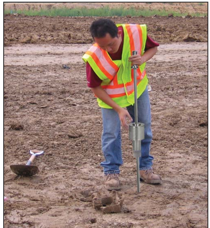
Dynamic cone penetrometer in use
