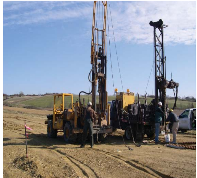
Soil boring and CPT testing of finished embankment
