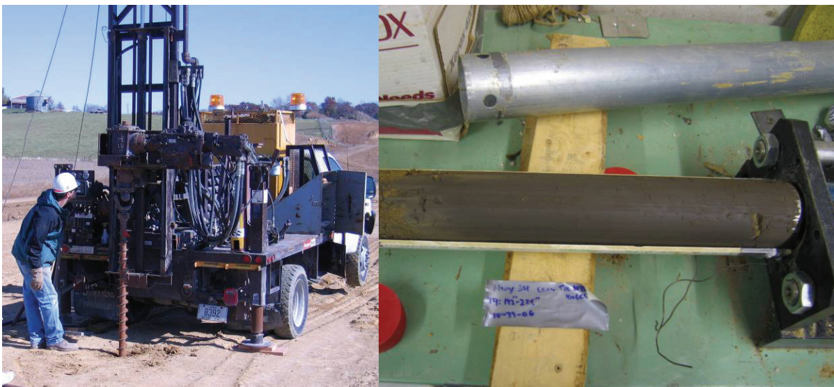
Figure 5. Shelby tube soil sampling in the field (right) and sample extrusion (right)
