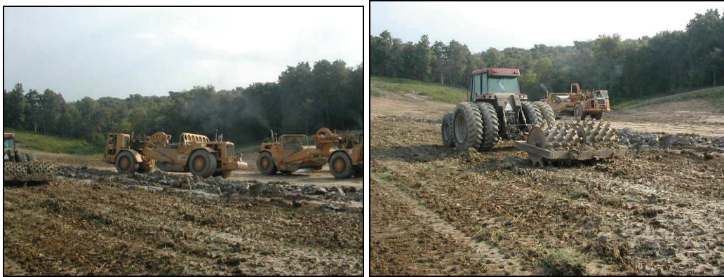
Figure 25. Scraper hauling soil and tractor-pulled sheepsfoot roller
