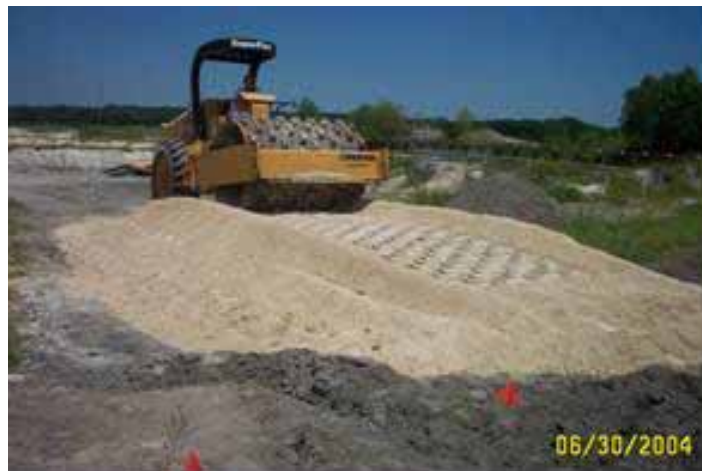
Figure 38: Compacting the test embankment
