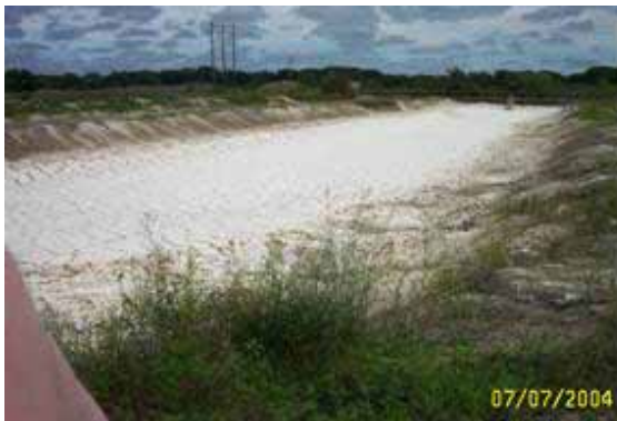
Figure 4: Dewatering lagoon after 10 months settling
