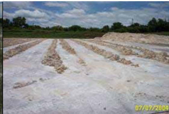
Figure 5: Solar drying of sludge in windrows
