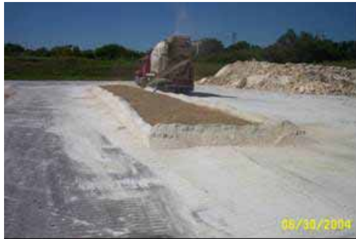
Figure 36: Pouring Fly Ash on a Lime Sludge Bed
