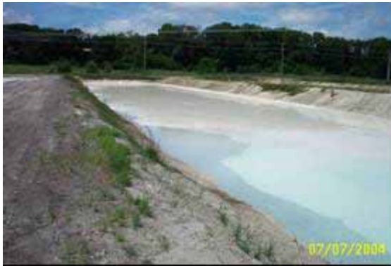
Figure 2: Dewatering lagoon while filling (looking towards the end from which the sludge enters)
