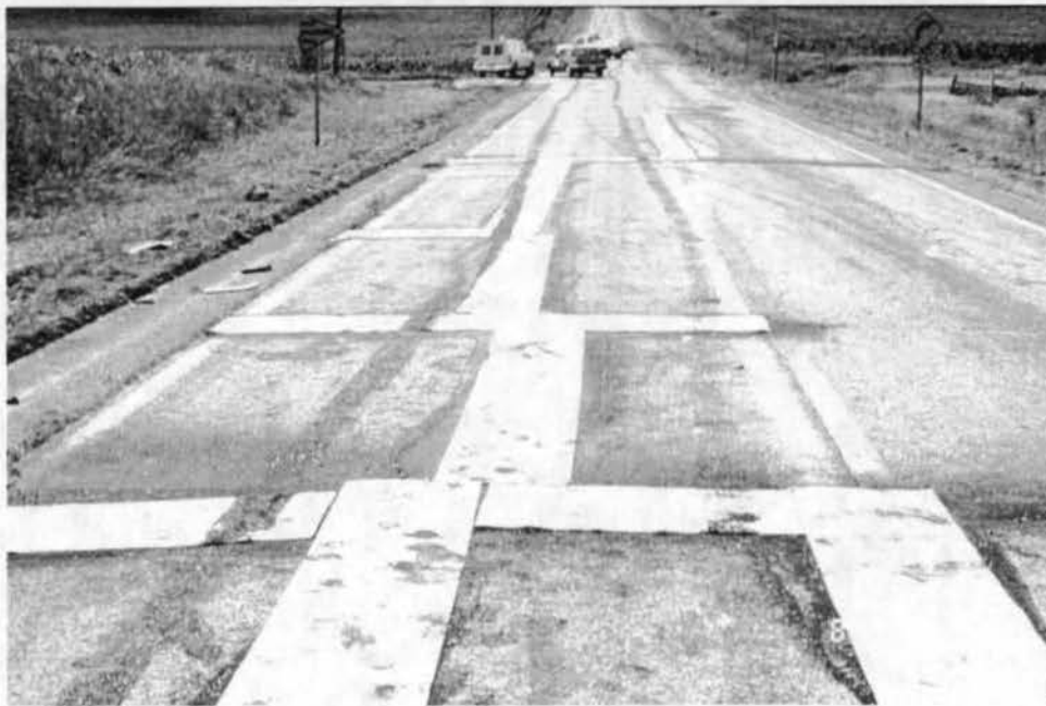
Placement of ProGuard fabric prior to spreading sand on exposed tack coat.
