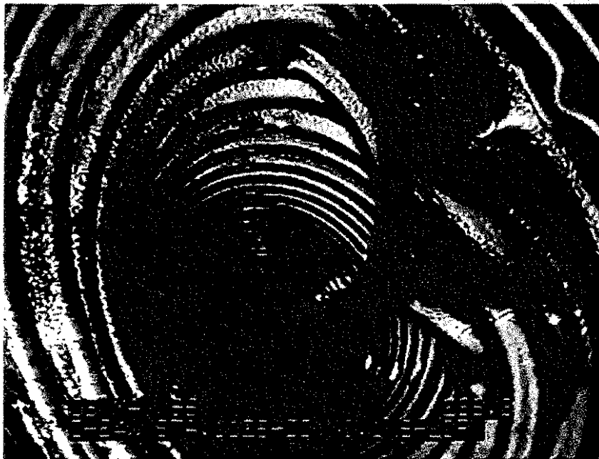
Figure 12. Crushed Mainline Segment at 238.3 Feet.
