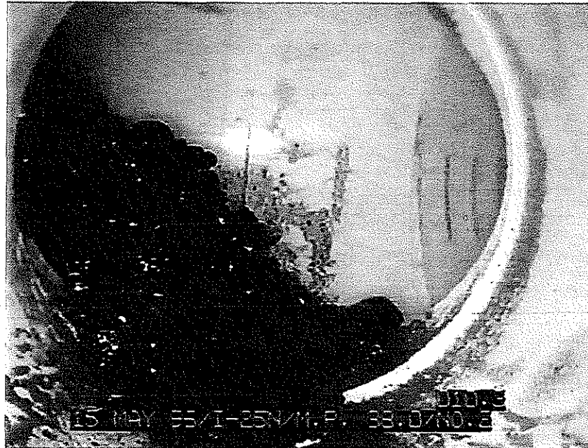
Figure 16. Asphalt-Stabilized Base in Edgedrain.
