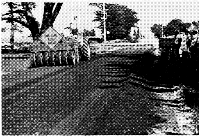
c. Rubber tired compaction.
