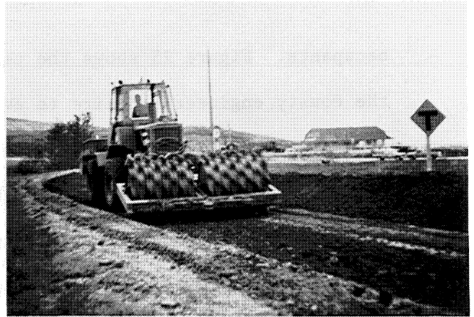
g. Tamping foot compaction, section N-2.
