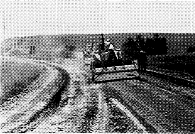
f. Rotary mixing, section N-2.
