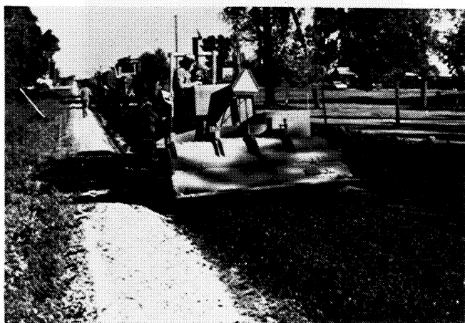
c. Rotary mixing, section HC-2.
