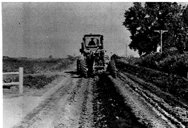
b. Initial blade grader mixing, section HC-2.
