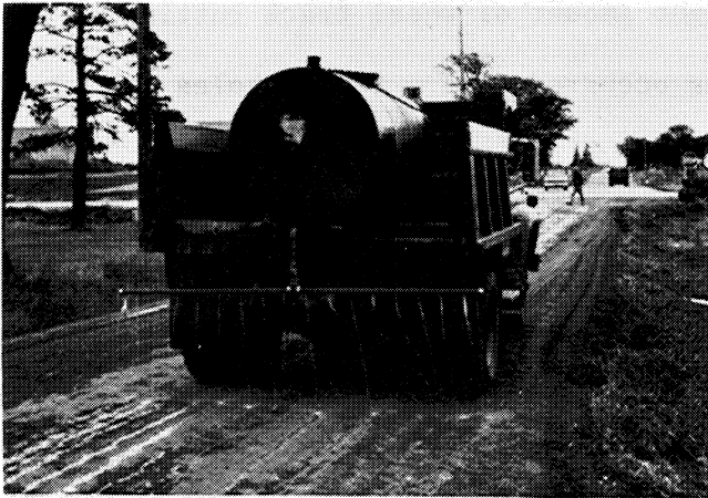
g. Second stage application of Coherex, October 16, 1980.
