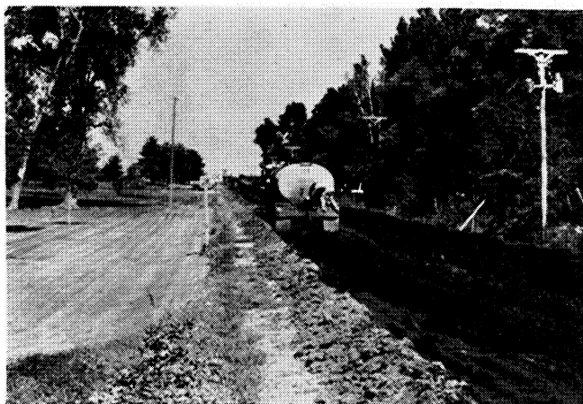
a. Asphalt emulsion application, section HC-2.
