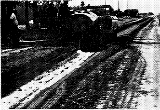
a. First stage application of Coherex to notched windrow.
