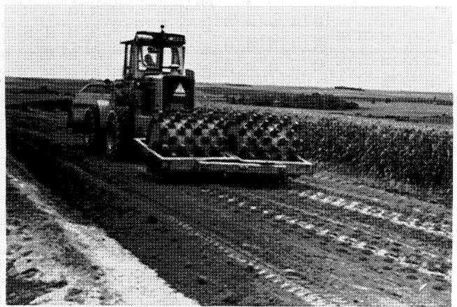
d. Tamping foot compaction.
