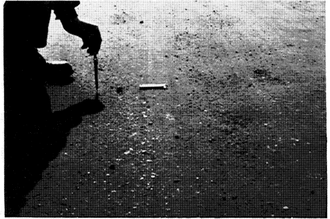
f. Exposed base course due to raveling of surface, February 28, 1980.
