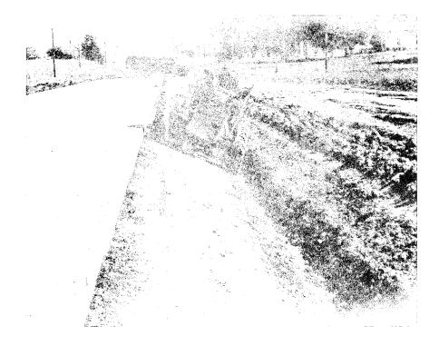
Photo 6: Cutting the 2:1 Shoulder Slope for the Styrofoam.
