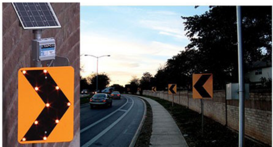
Figure 1. Sequential dynamic curve warning system (FHWA 2012)
