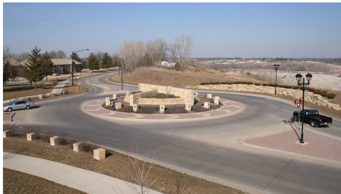
Figure 6. Example of horizontal displacement (roundabout) (Hillary Isebrands/Institute for Transportation)
