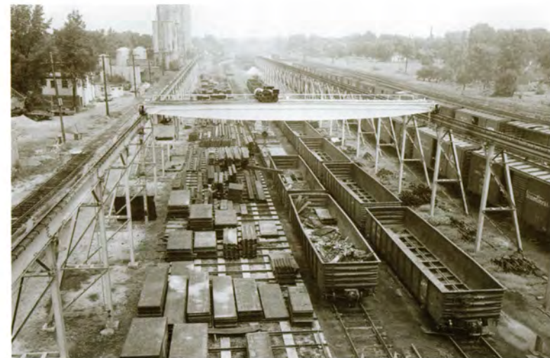
The Overhead Crane
