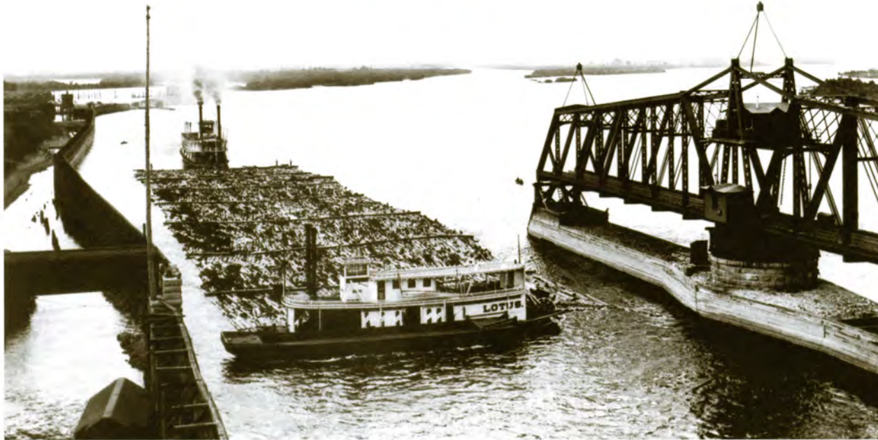
The C&NW draw span open to permit passage of a lumber boom in the west channel, ca. 1900.
