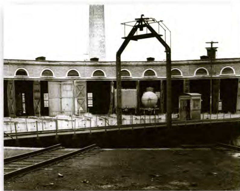
The abandoned roundhouse at the Camanche Avenue yards, ca. 1970
