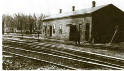
The Road House, ca. 1910.
