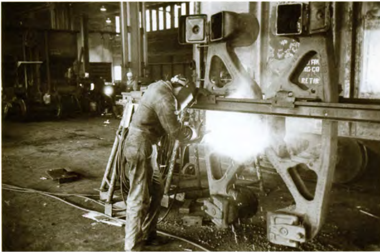
Welding in the Car Shops
