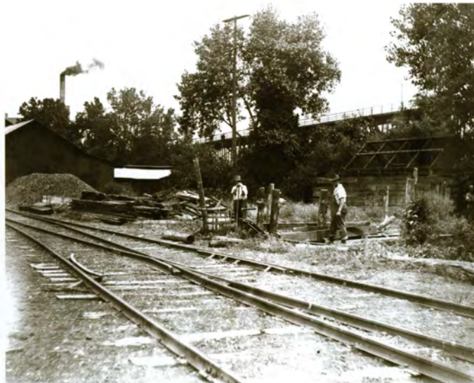
Workmen at railside in the Lyons yards, 1916
