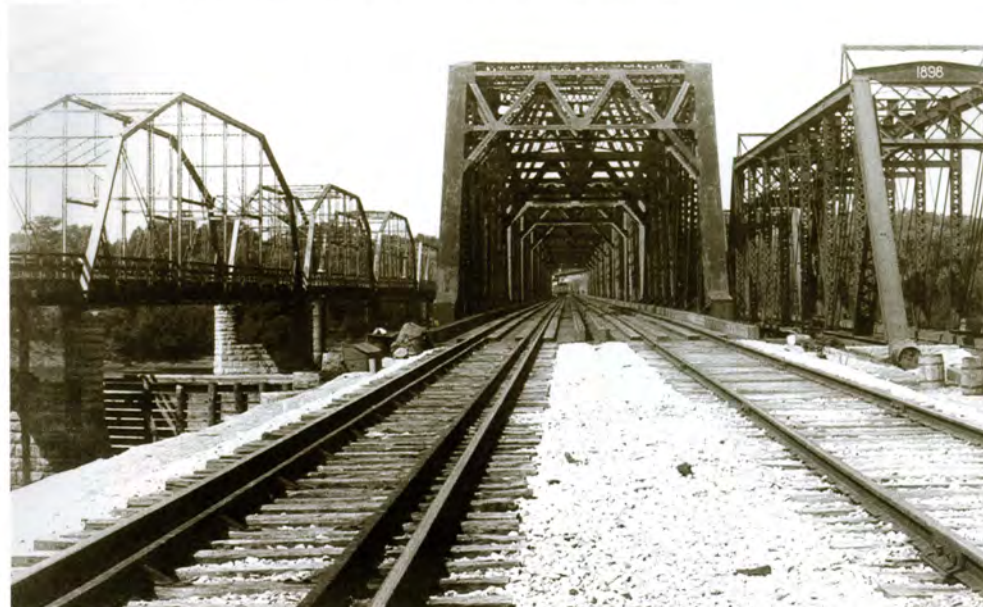
The 1898 and 1909 Chicago & North Western bridges side by side with the High Bridge, ca. 1909
