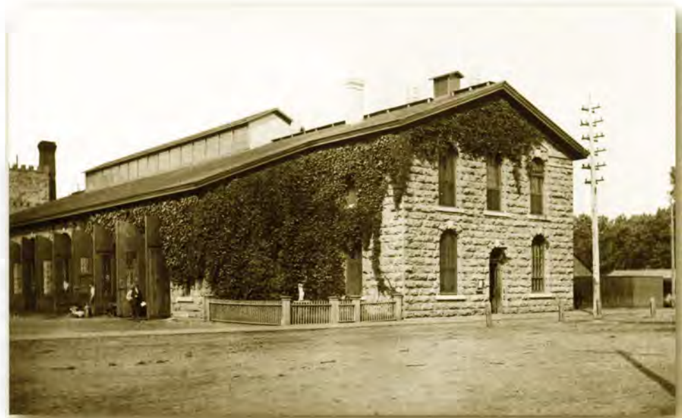
The Chicago & North Western machine shop at the old yards downtown, ca. 1885.
