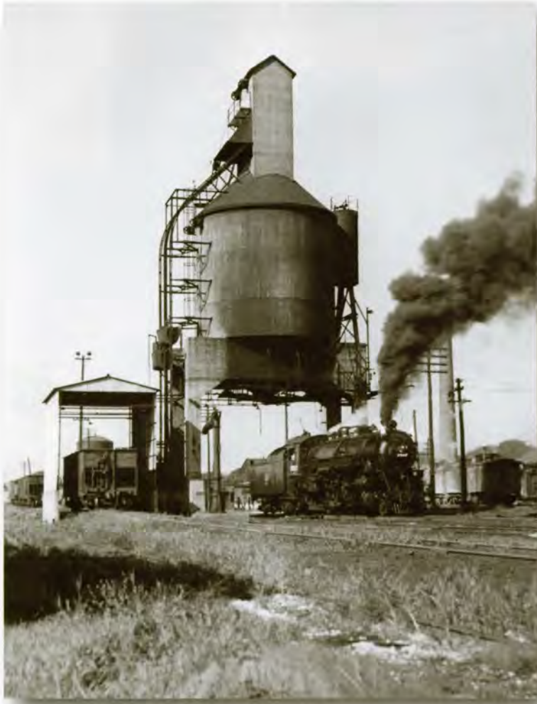
Loading coal at the new Camanche Avenue yards.
