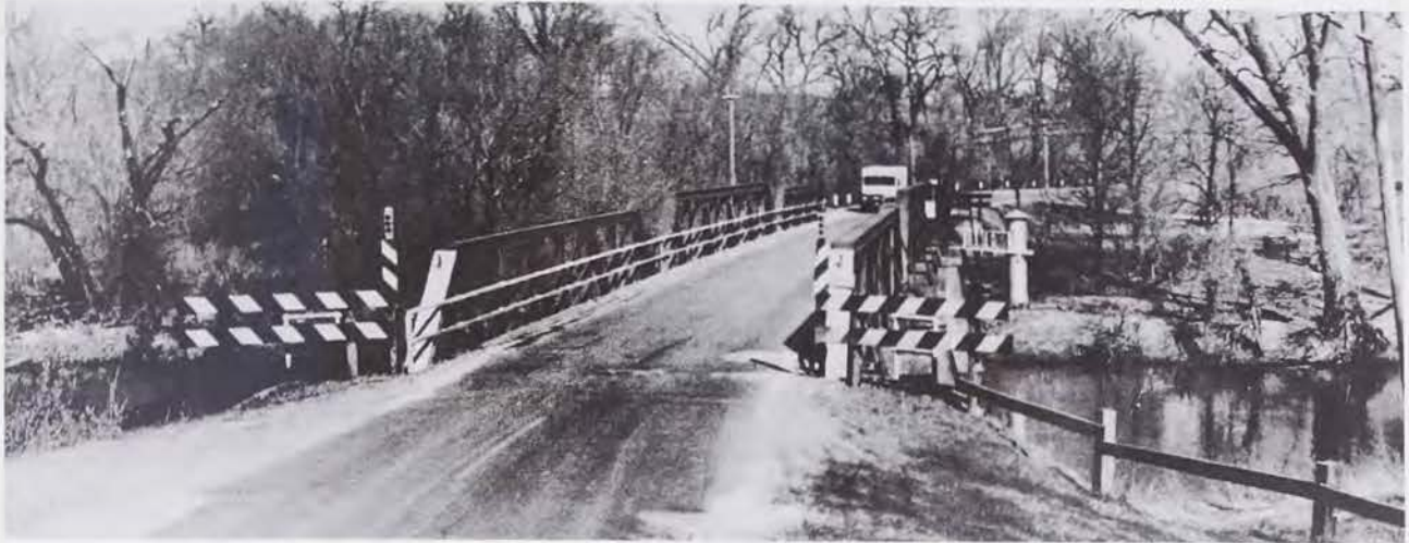
An inadequate primary road bridge typical of the bridge problem that existed in the early 1960s. (Courtesy: Iowa State Highway Commission)
