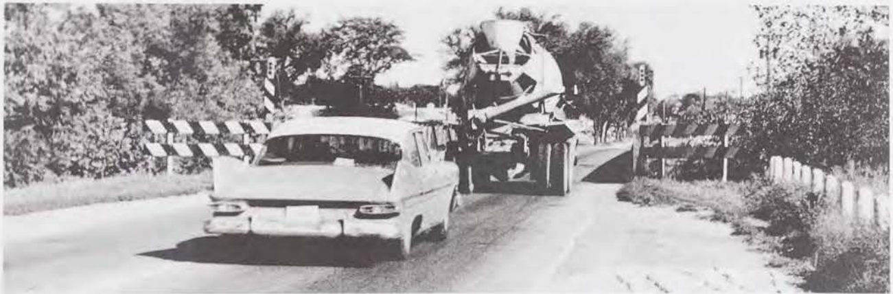
Inadequate roads and bridges typical of the state primary road system in the 1950s. (Courtesy: Iowa Highway Needs Study 1960-1980)
