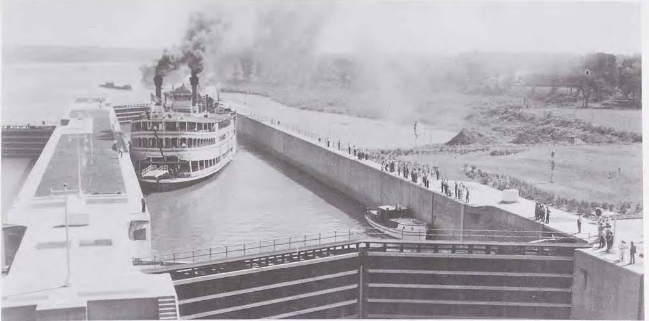
Mississippi River Lock & Dam No. 15. Naval Reserves boat and Str. J.S. locking through, 1933. (Courtesy: U.S. Army Corps of Engineers, Rock Island District)
