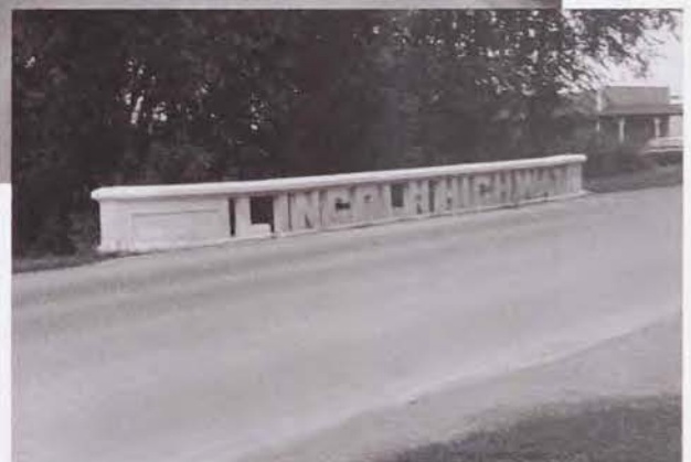
Bridge at Tama on old road, 1986. (Courtesy: Author)
