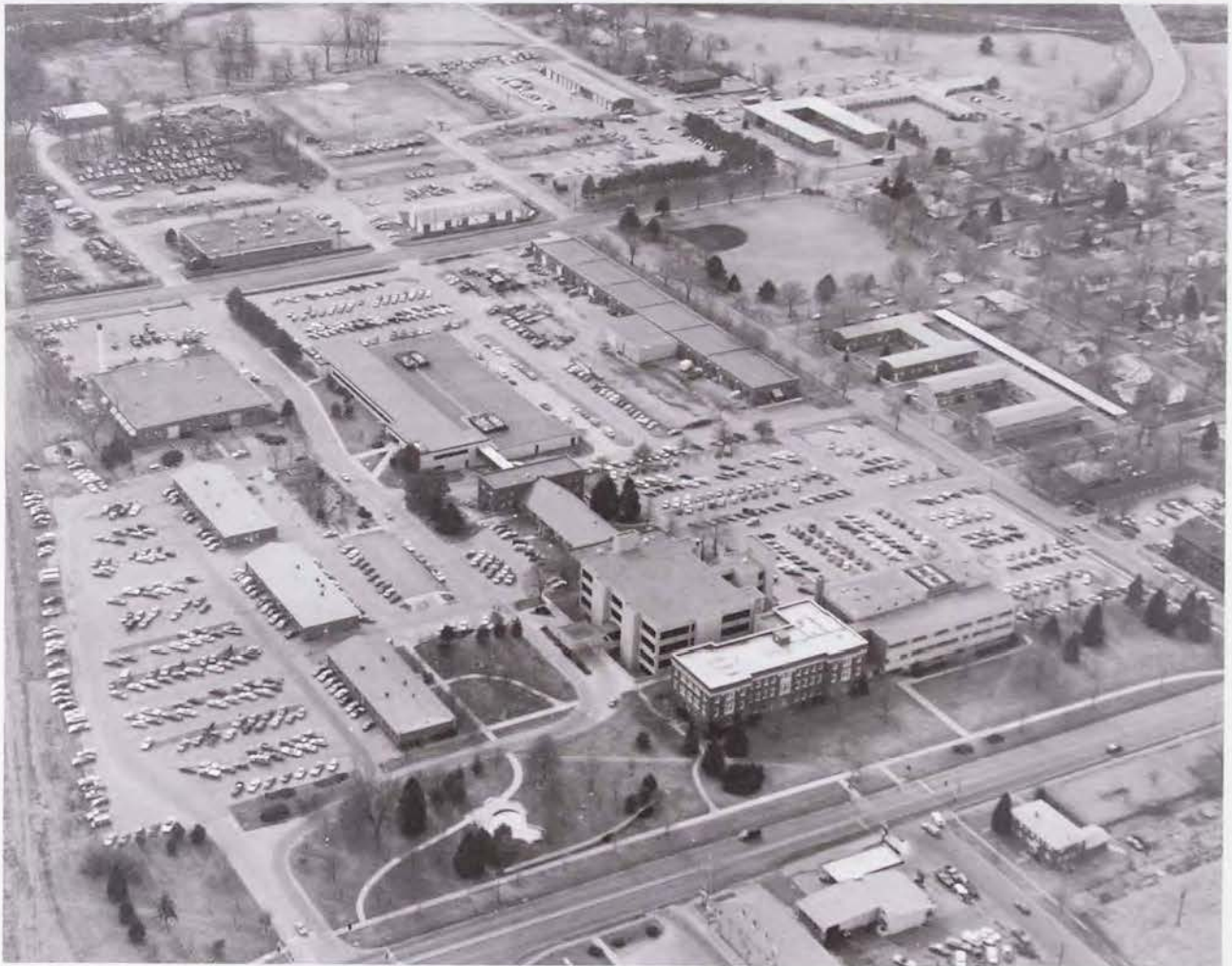
Aerial view of Department of Transportation's Ames complex in 1986. (Courtesy: Iowa Department of Transportation)
