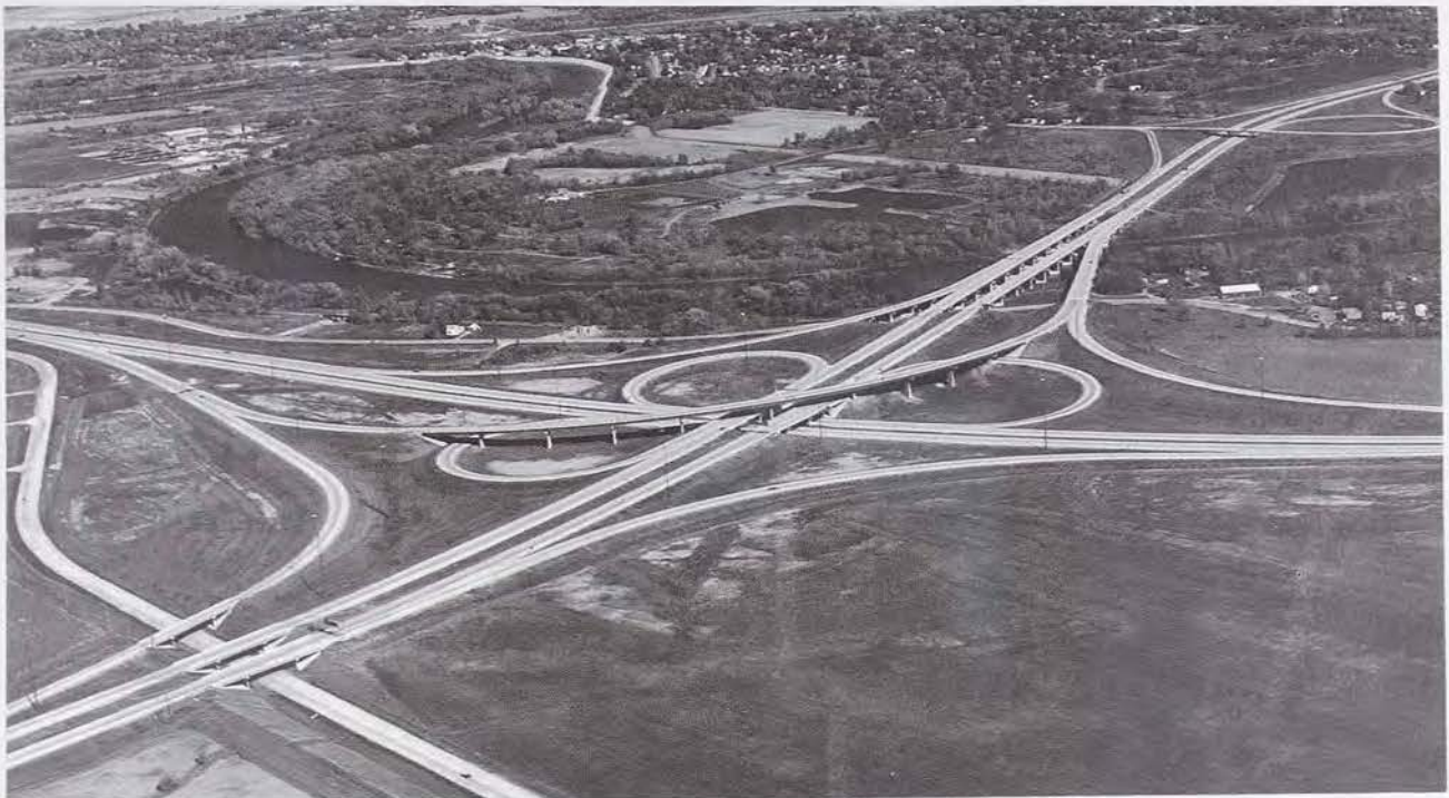
Interchange of Interstate 380, U.S. 20 and U.S. 218 at southeast corner of Waterloo. (Courtesy: Iowa Department of Transportation)
