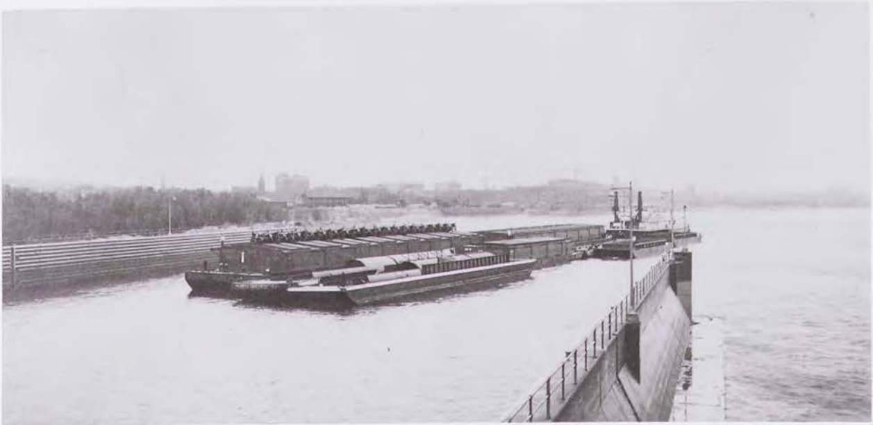
Mississippi River Lock No. 15. Federal Barge Line steamer Mark Twain with tow entering main lock, 1936. (Courtesy: U.S. Army Corps of Engineers, Rock Island District)
