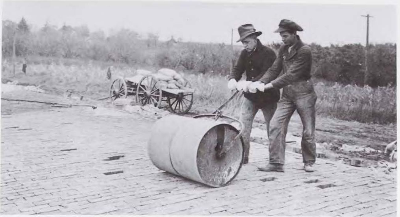
Rolling the Des Moines to Camp Dodge brick pavement with a 700 pound roller, 1917-1918 (Courtesy: Iowa State Highway Commission)
