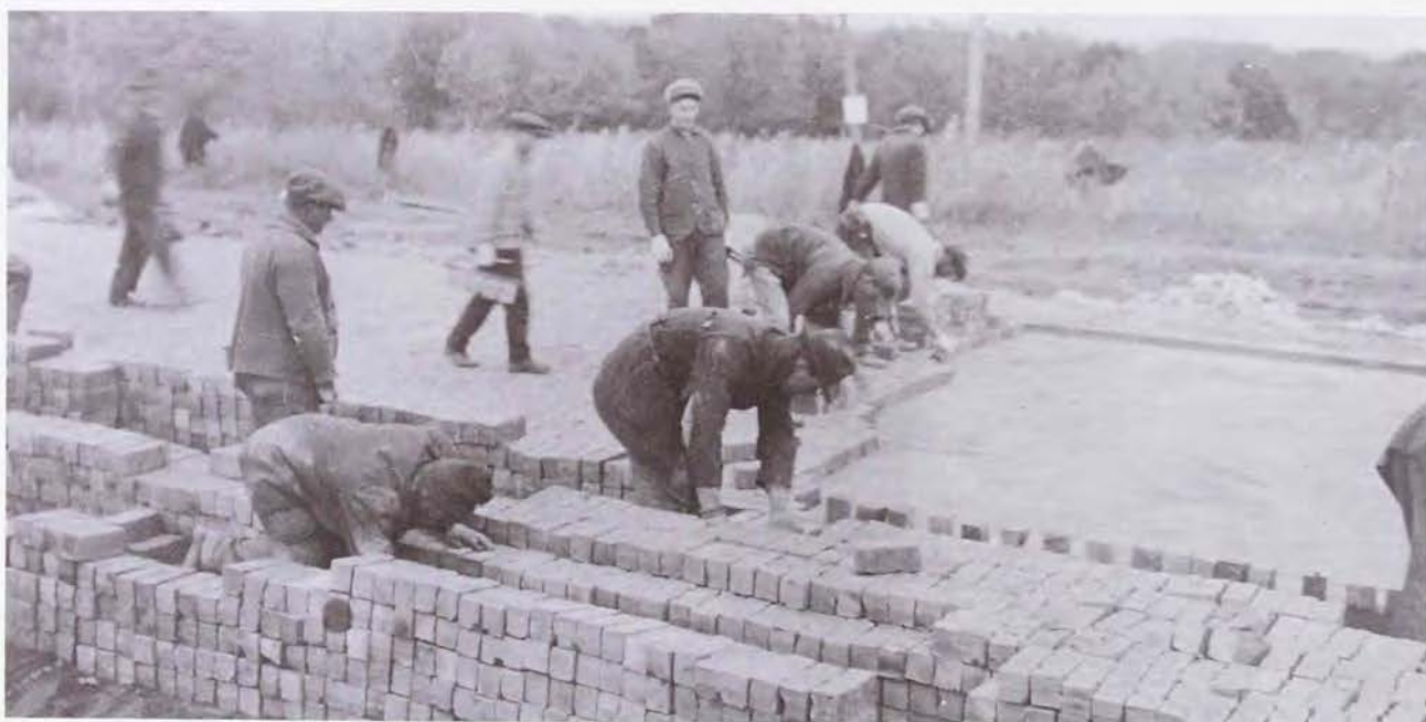
Placing monolithic brick pavement for the Des Moines to Camp Dodge road, 1917-1918. (Courtesy: Iowa State Highway Commission)
