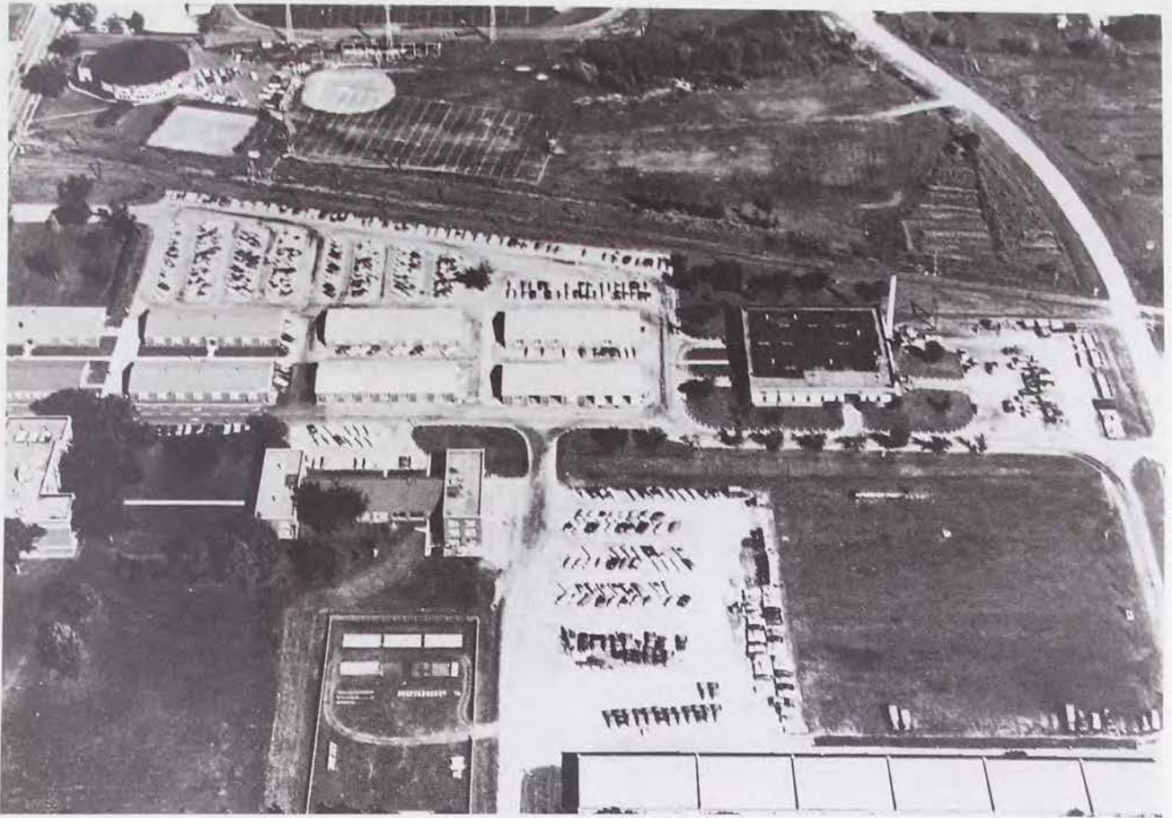
Aerial view of Highway Commission's Ames complex in the 1950's. (Courtesy: Iowa State Highway Commission)
