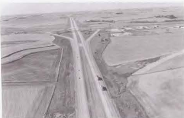
Interstate 80 in Iowa. (Courtesy: Iowa Department of Transportation.)
