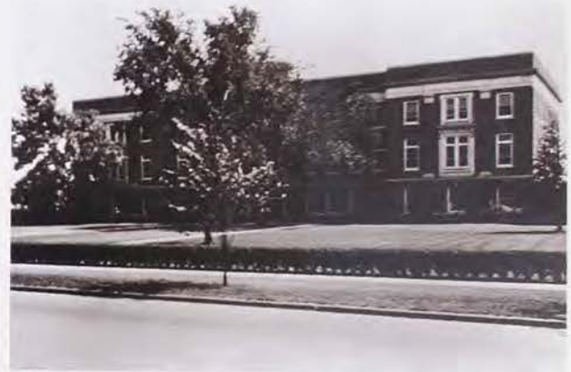
The original Highway Commission building completed in 1923. (Courtesy: Iowa State Highway Commission)
