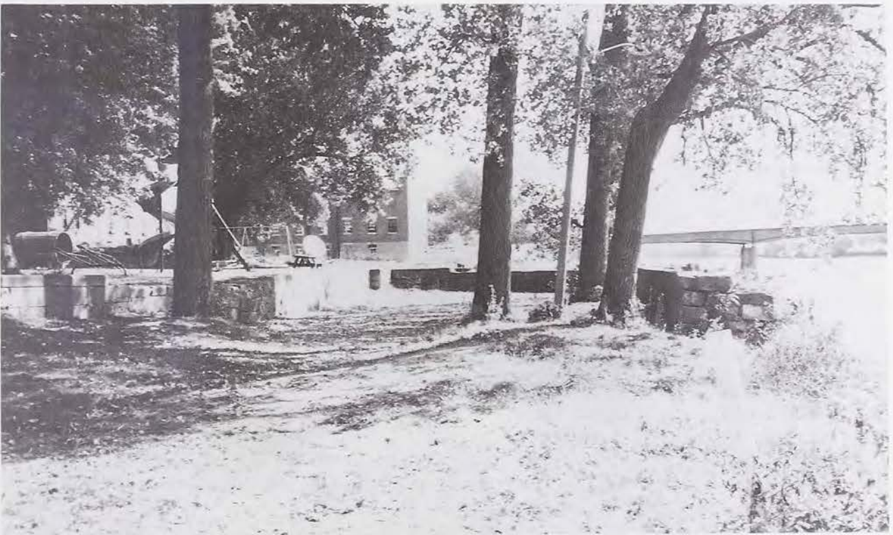
Remnants of the Dam and Lock at Bonaparte.
