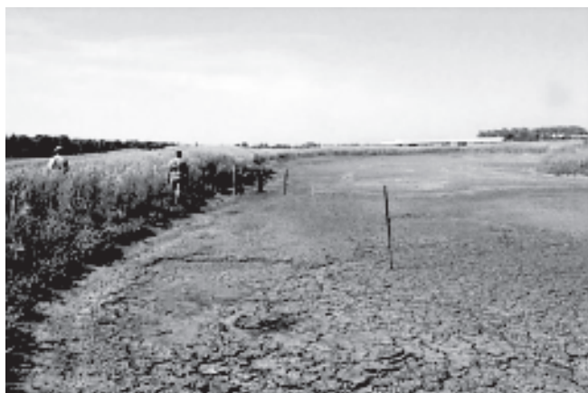
Dewatered solid settling basin below beef feedlot.
