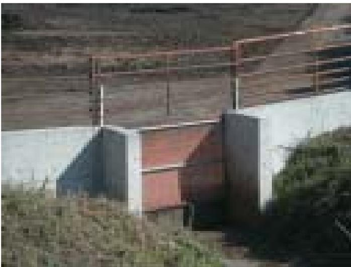
Solids settling basin on feedlot with less than 1,000 animal units.
